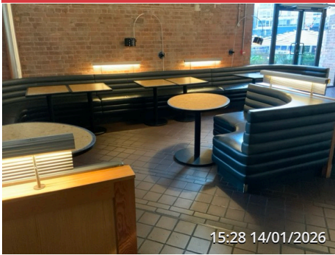
ITEM 7 STRIP OUT BOOTH SEATING
