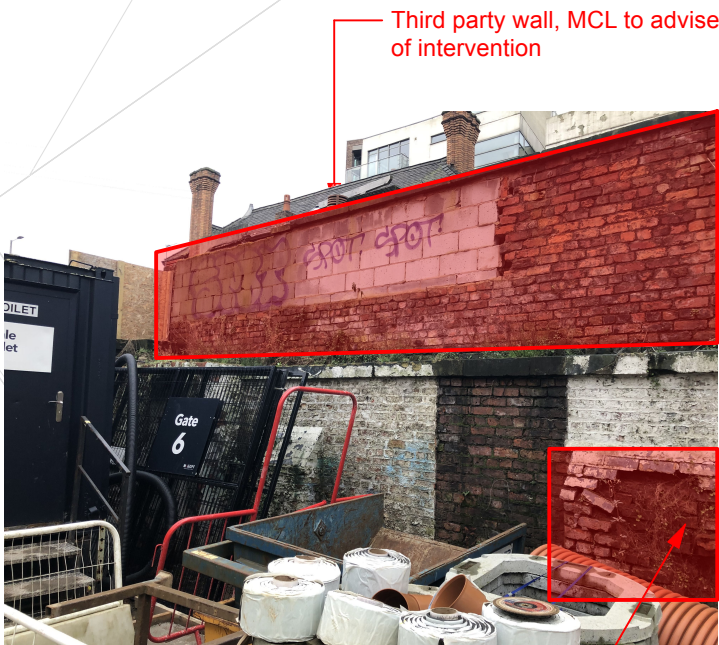
Wall D - Existing condition
