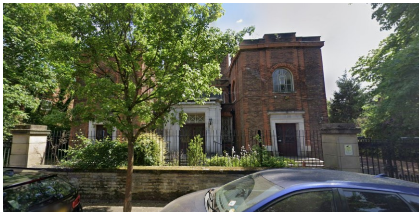
Figure 4. The Synagogue of Withington on Old Lansdowne Road – Google Street View
