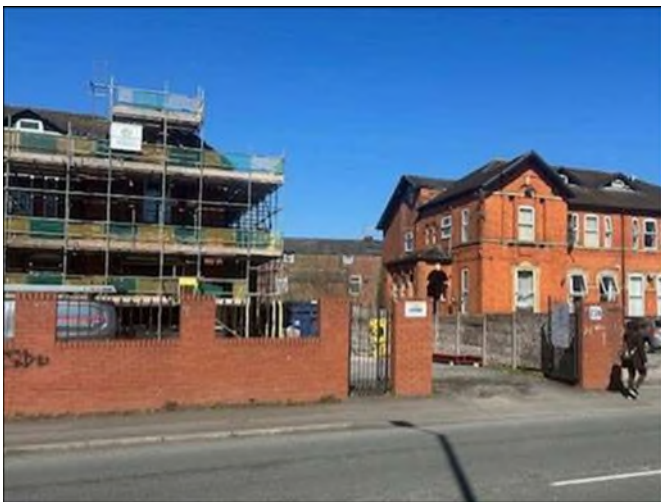
Application property presently enclosed by scaffolding.
