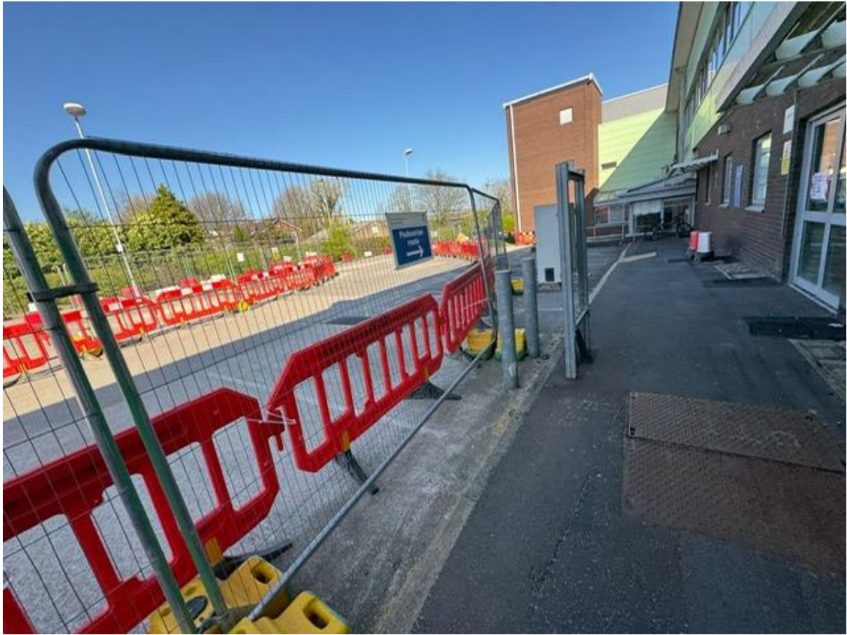
SITE PHOTOS MAY 2025
