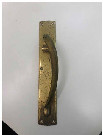
Existing Pull Handle - use least tarnished and clean to same standard as window stays Door Suite: 5
