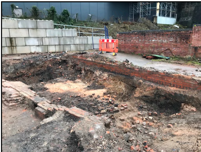
Plate 2.1: Chapelfield Dye Works Excavation
