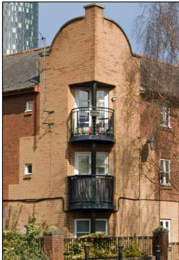
Corner View – Chorlton Road / Eliza Street (View B)
