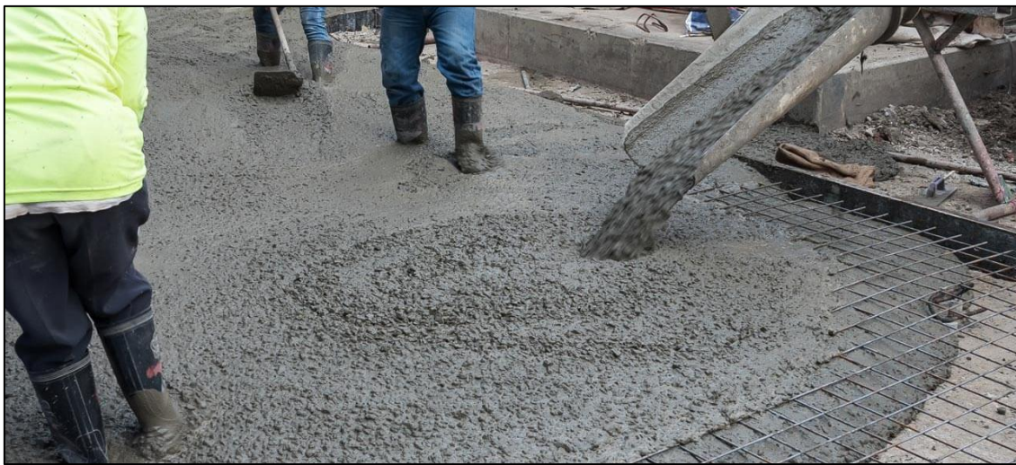
Figure 2. Pour of concrete slab. Where cement replacement and minimisation practices are implemented the carbon impact associated with concrete elements can be notably reduced.
