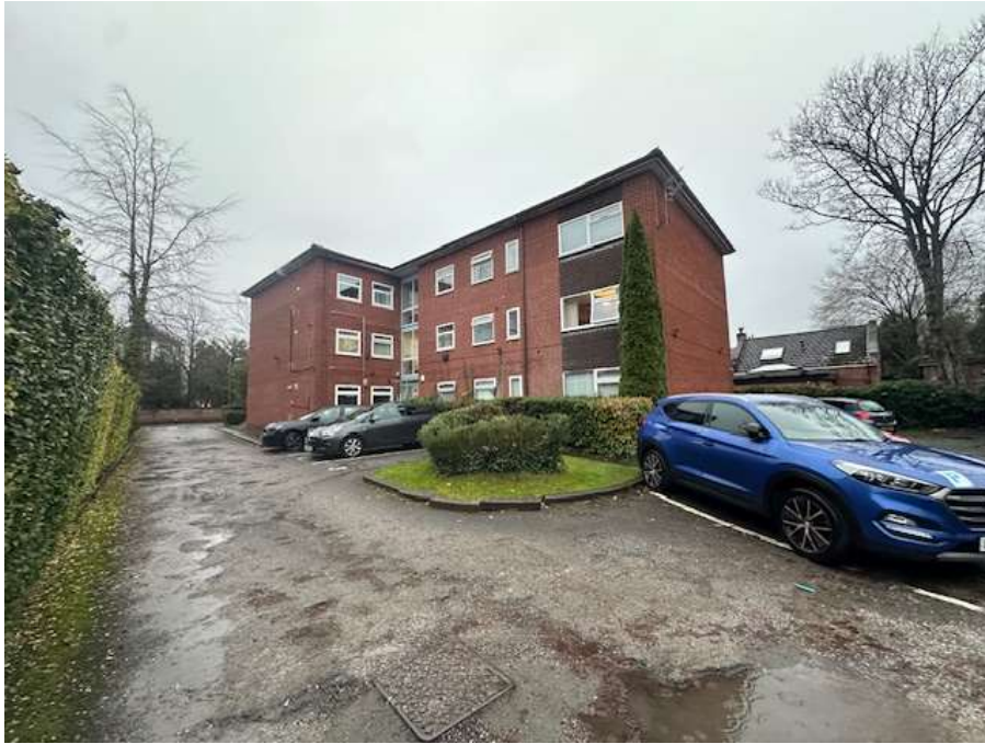
Figure 2: Side/rear elevations of the application property when viewed from NW (site resident carpark/bin store).
