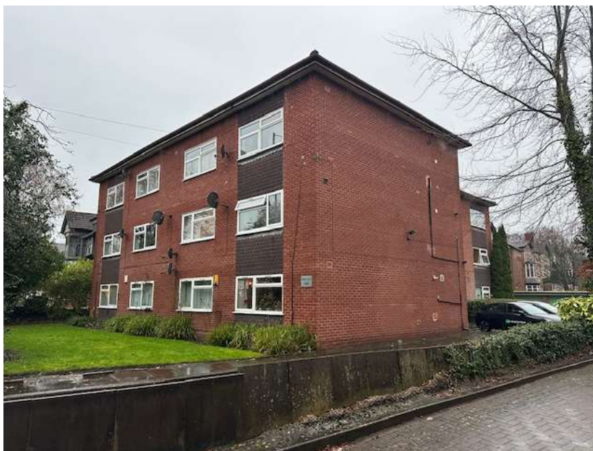
Figure 1: Principal elevation of the application property - Balholm Court.
