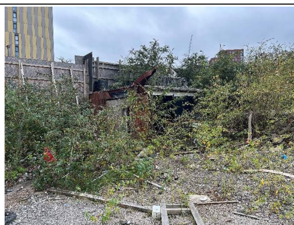
2. Retained structure in the south of site (photo looking SW)
