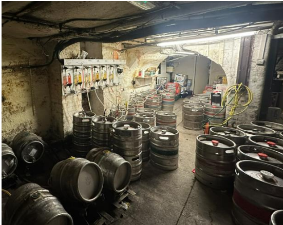
E. Basement, view from staircase.
