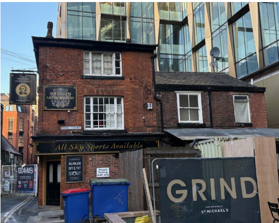
F. East Facade from Bootle Street, taken in January 2026
