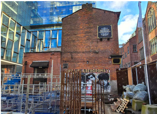
D. West Facade from within No.02 St Michaels, taken in January 2025
