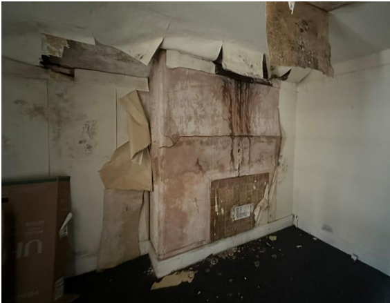
E. Second Floor Room 02
