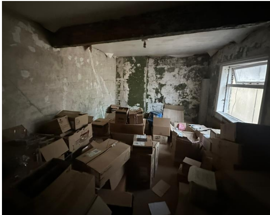
D. Second Floor Room 01
