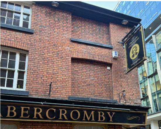
C. Bootle Street Historic Fenestration - Current Infill
