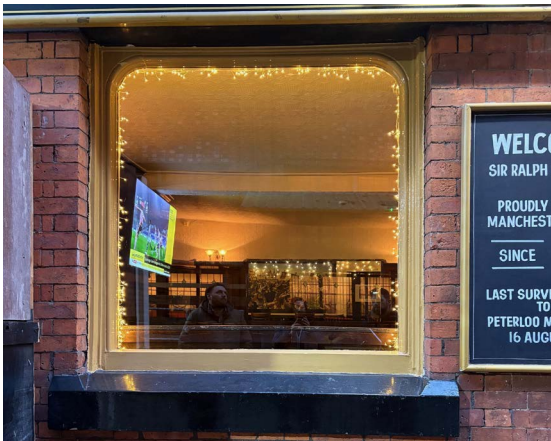
A. Bootle Street Ground Floor Fenestration
