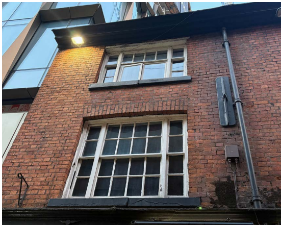
B. Bootle Street Upper Floor Fenestration
