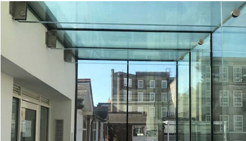
Structural Glass Box with structural glass fins - design intent
