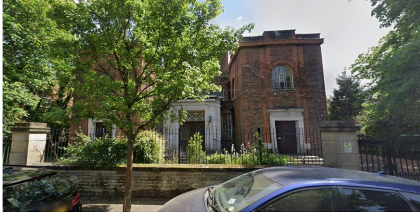
Figure 5. The Synagogue of Withington on Old Lansdowne Road – Google Street View
