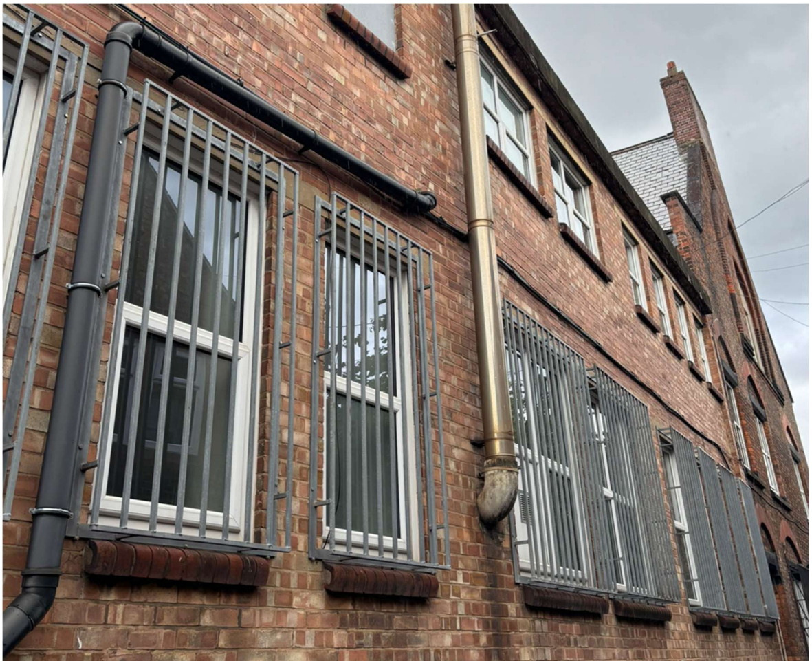
Figure 5 – Existing security grilles
