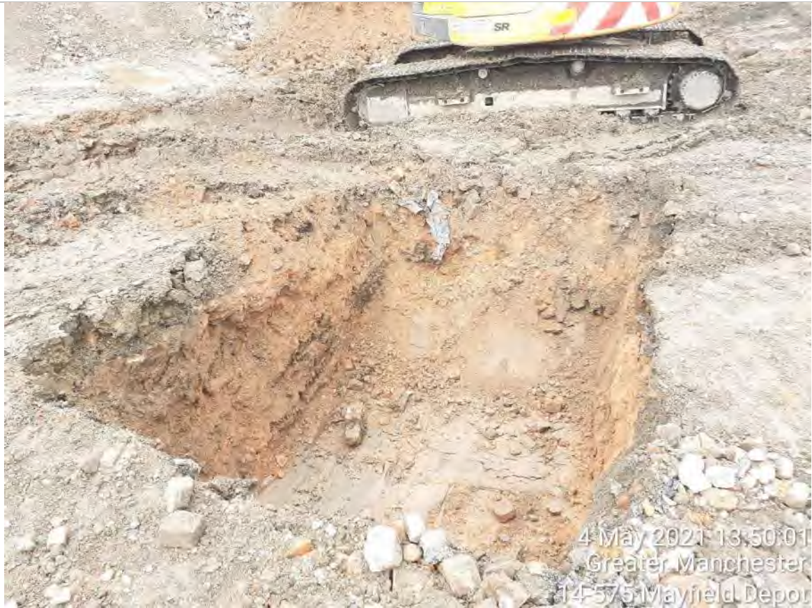
PLATE 7 TP103 HOTSPOT REMOVAL
