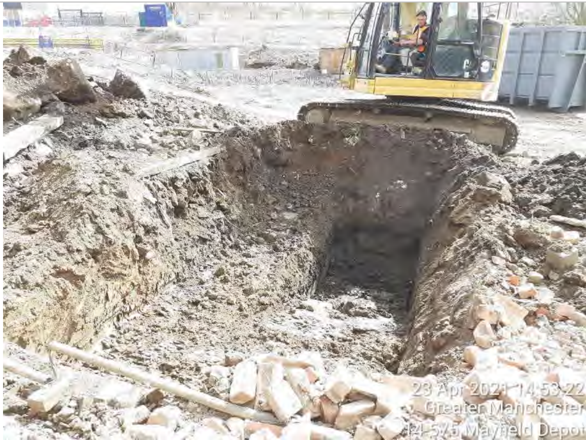
PLATE 4 TP302 HOTSPOT REMOVAL
