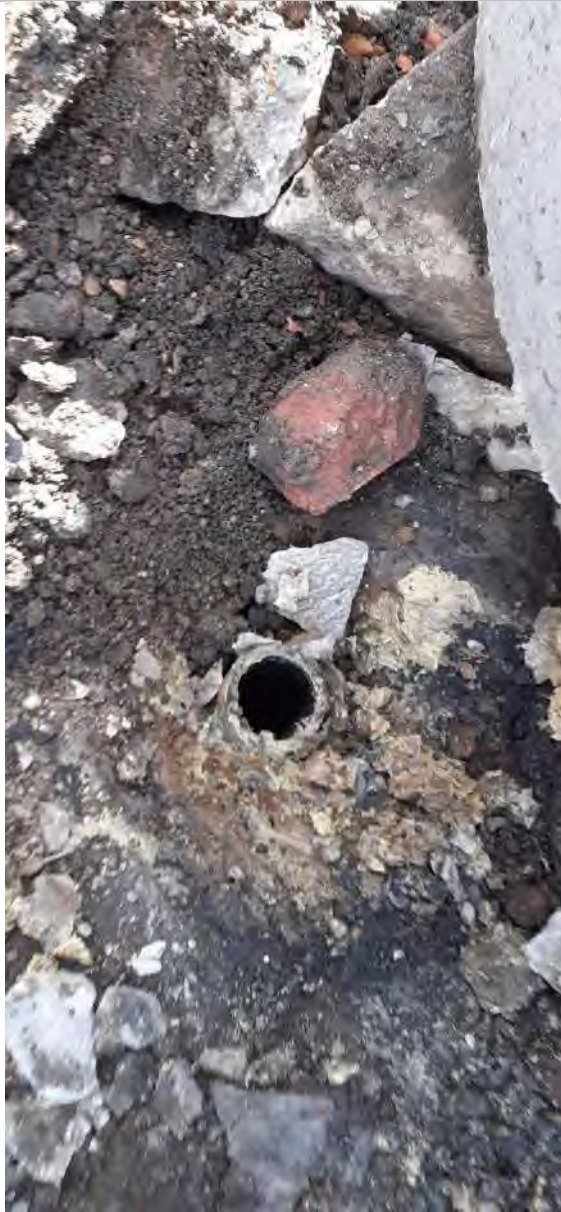
PLATE 12 GROUTING OF MONITOURING WELLS
