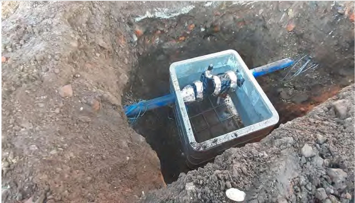
PLATE 14 PROTECA-LINE BARRIER PIPE FOR WATER SUPPLY PIPEWORK.
