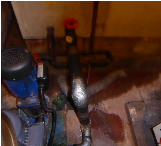
Main Roof Void Bay 1
