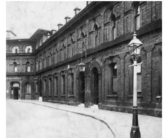
— C - View south from Baring St.
