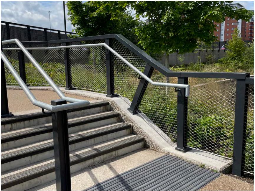
—Steps To match steps within Mayfield Park.
