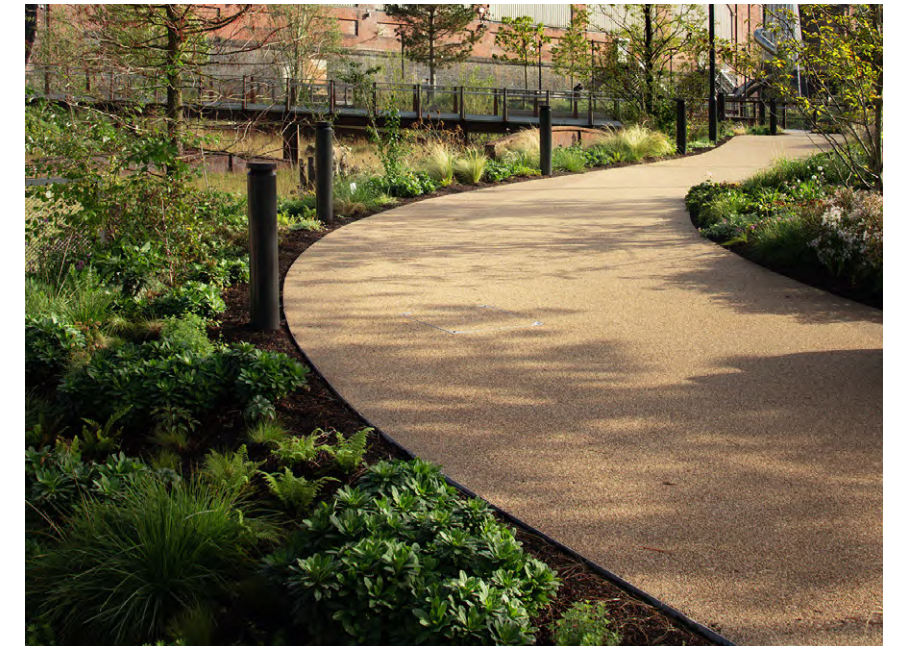
—Positive falls to planting Allowing the opportunity for all impermeable surfaces to fall towards soft landscaping
