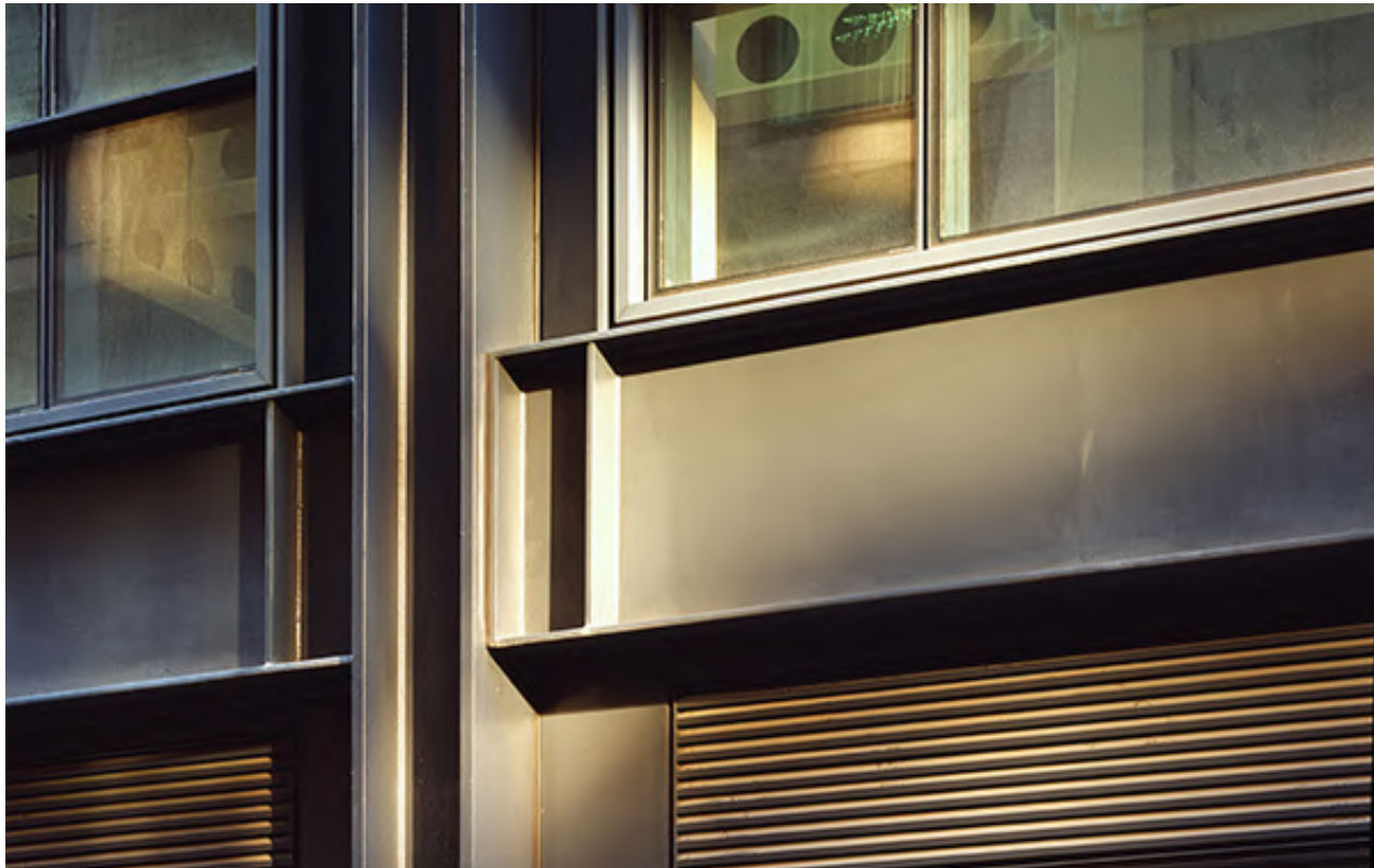
—Industrial facade photograph Devonshire Square, London.
