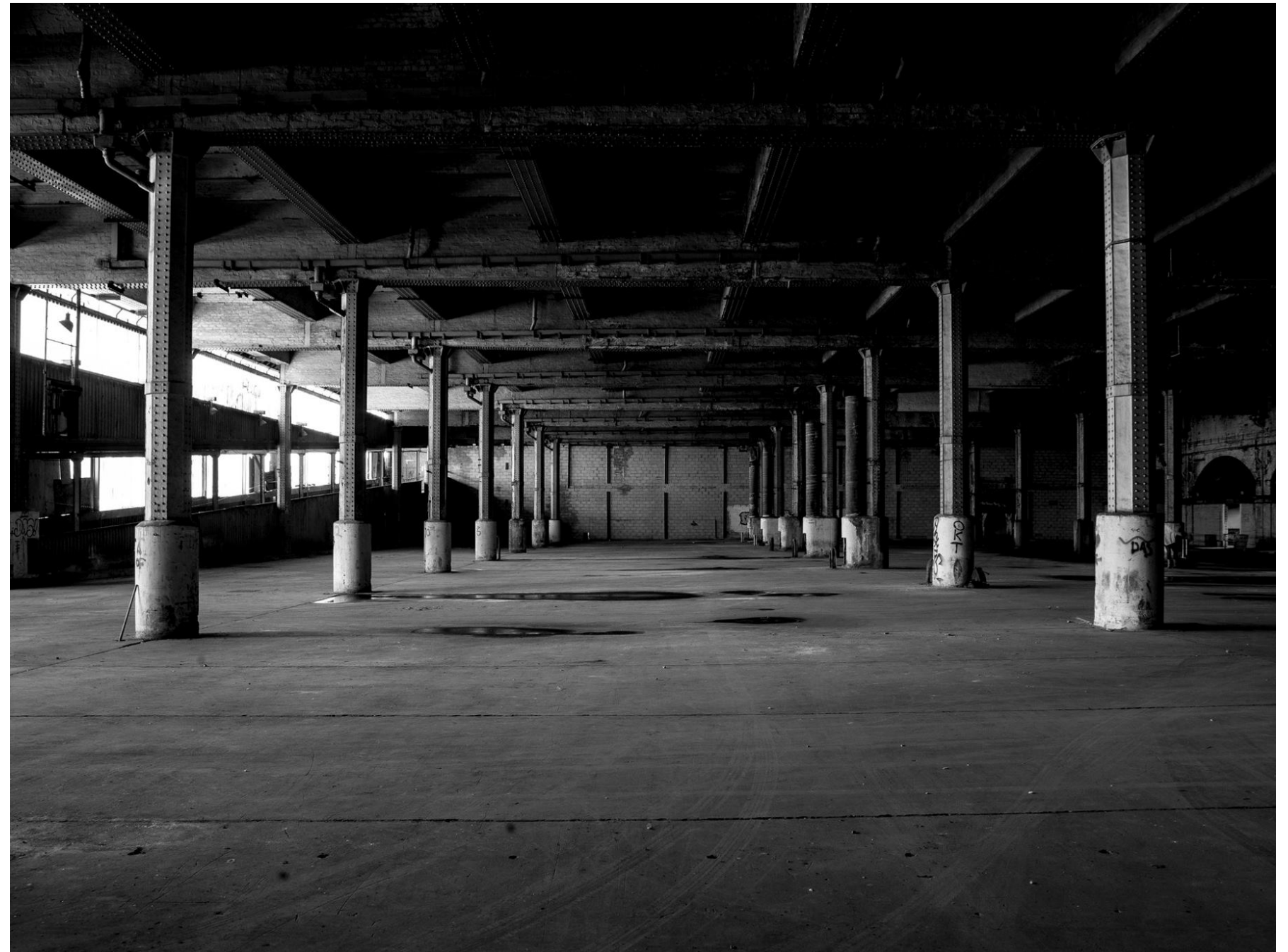
—Mayfield depot Interior photograph of expressed structural frame.
