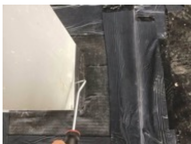
Probe testing stanchion detailing
