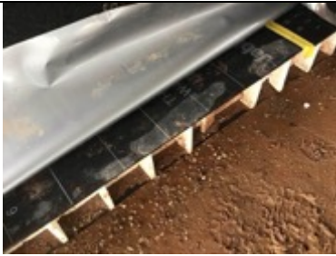
Heave board installed which the membrane is installed above
