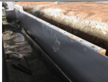
Membrane extended up the perimeter shuttering
