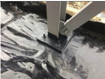
Sealed stanchion detailing
