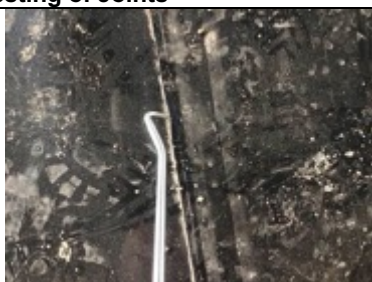
Probe test to auto welded membrane lap joint
