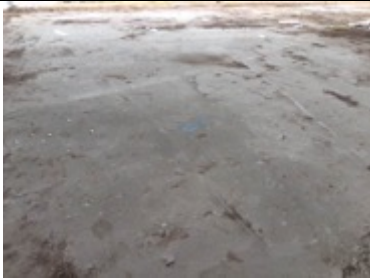
Sand blinded well rolled and compacted
