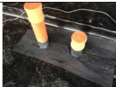
Sealed pipe penetrations
