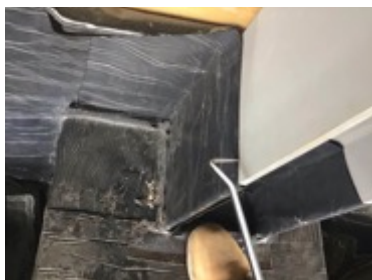
Probe testing stanchion sealing
