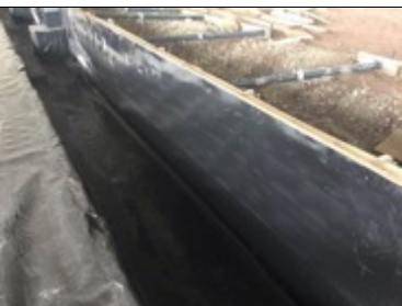
Membrane extended up the internal perimeter shuttering
