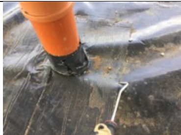
Pick testing to the pipe detail to Pour area 3.
