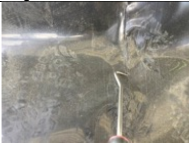
Pick testing to the hand welded Lap joint within pour area 3.
