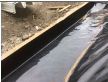
Membrane extended up the perimeter temporary shuttering
