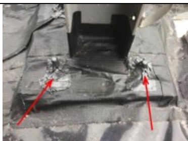
Butyl tape used to seal bolts
