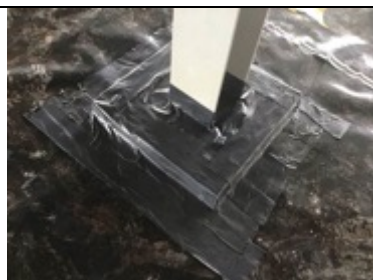
Sealed stanchion detailing
