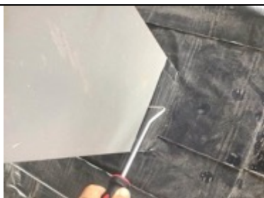
Probe testing stanchion detailing
