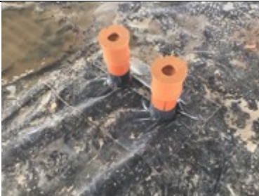
Sealed pipe penetrations
