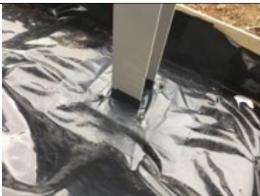
Sealed stanchion detailing
