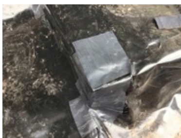
Sealed corner detailing
