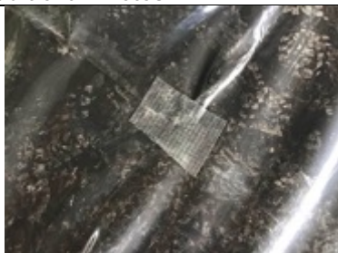
Defect repaired sealed using Juta GP1 SAM
