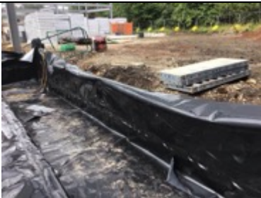
Perimeter membrane extended over the temporary shuttering
