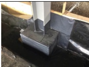
Sealed internal stanchion and concrete surround detailing
