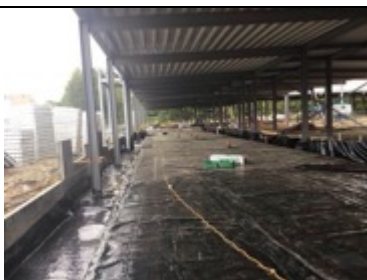
Pour 3 overview of completed works
