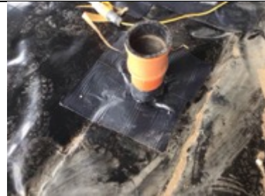
Sealed pipe penetrations
