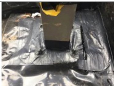
Sealed stanchion detailing
