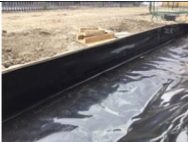
Membrane returned up the perimeter shutter and stapled at the top into place.
