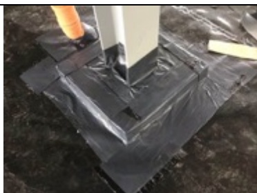
Sealed stanchion detailing
