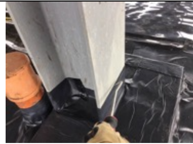
Pick testing to the stanchion detail within pour area 5.
