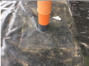
Sealed pipe penetration detail within pour area 3.
