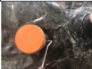
Probe testing pipe sealing
