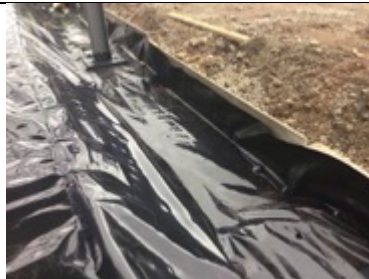
Perimeter membrane extended up the shuttering
