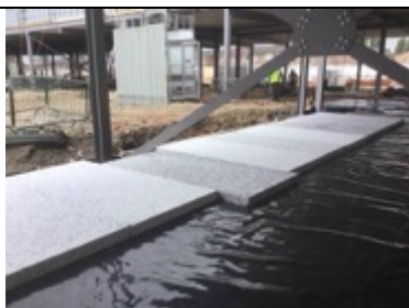
Insulation installed after the inspection
