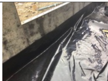
Membrane extended up the outer perimeter shuttering
