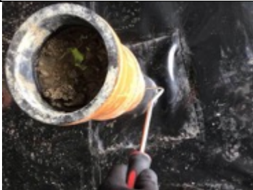
Testing Juta GP1 SAM sealing the top hat to the pipe sleeve
