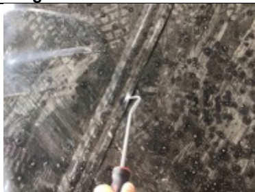
Testing auto welded membrane lap joint
