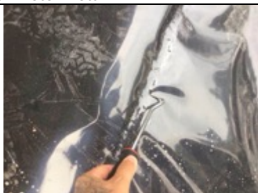
Testing perimeter membrane hand welded lap joint
