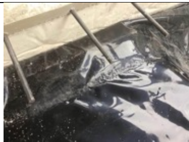
Membrane hand welded to the existing membrane from pour 1b
