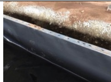
Membrane extended up the perimeter shuttering
