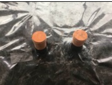
Sealed pipe penetrations
