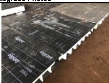
Heave board installed prior to the membrane installed above
