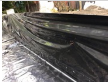
Perimeter membrane extended over the temporary shuttering
