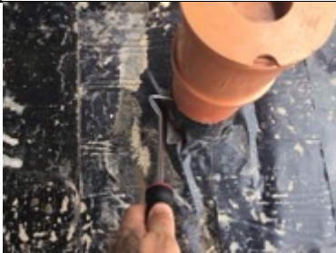
Testing pipe seals
