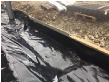
Perimeter membrane extended up the shuttering
