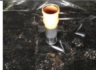
Pipe penetration sealed using hand welded preformed top hat and Juta GP1 SAM
