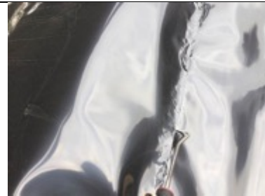
Pick testing carried out along the hand welded lap joint to pour area 5.
