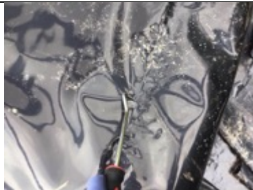
Testing sealed hand welded membrane lap joint
