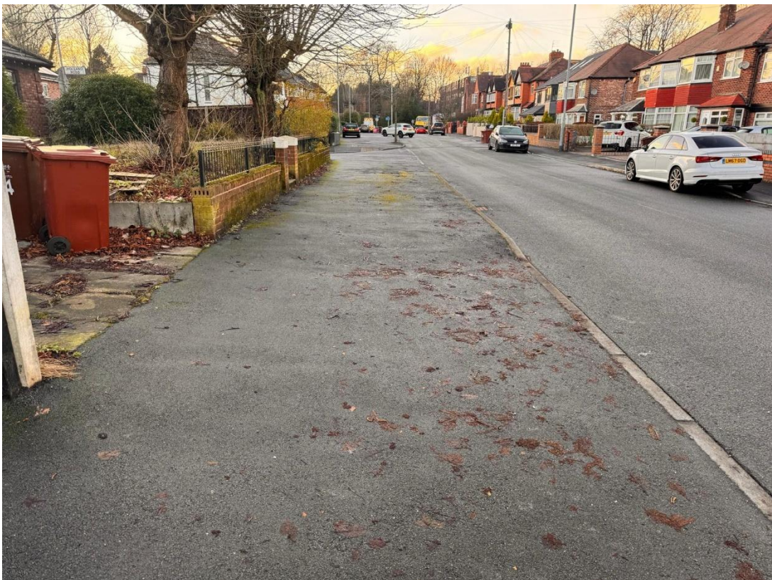
Figure 2: Pavement adjacent to Wilton Road, facing west.
