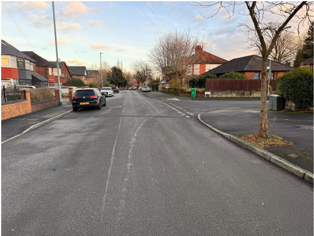
Figure 7: Junction between Wilton Road and Holland Road, facing east.
