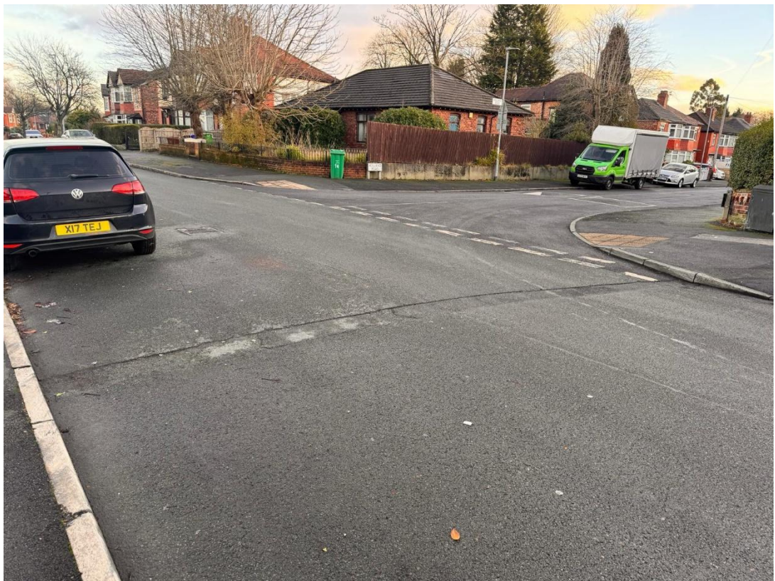
Figure 8: Junction between Wilton Road and Holland Road, facing south-east. This pictures the existing trench reinstatement on Wilton Road.
