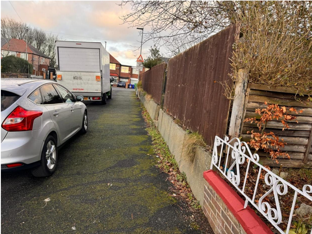
Figure 9: Pavement adjacent to Holland Road, facing north. This portrays the existing moss growth on the pavement.
