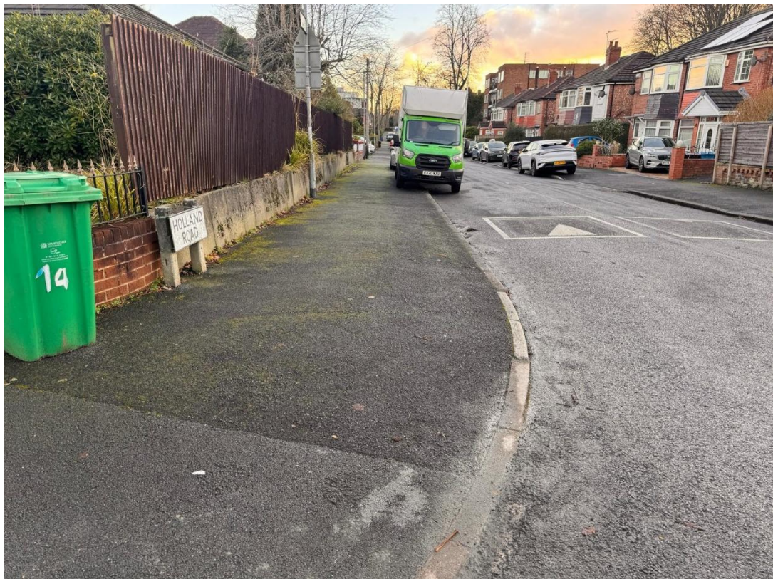
Figure 6: Pavement adjacent to Holland Road, facing south.
