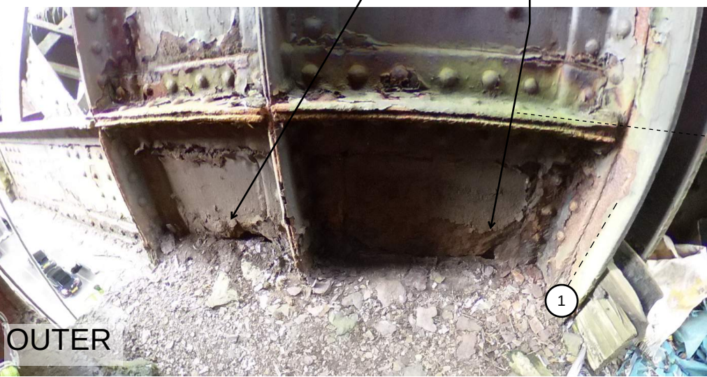
Holes to bottom of lower panels
