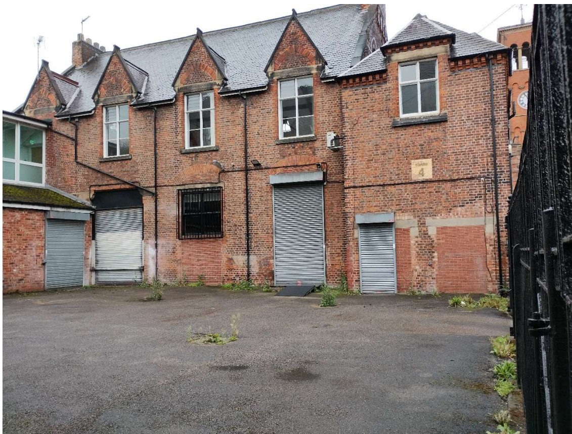
Figure 2 Courtyard showing ramp into south wing of the building
