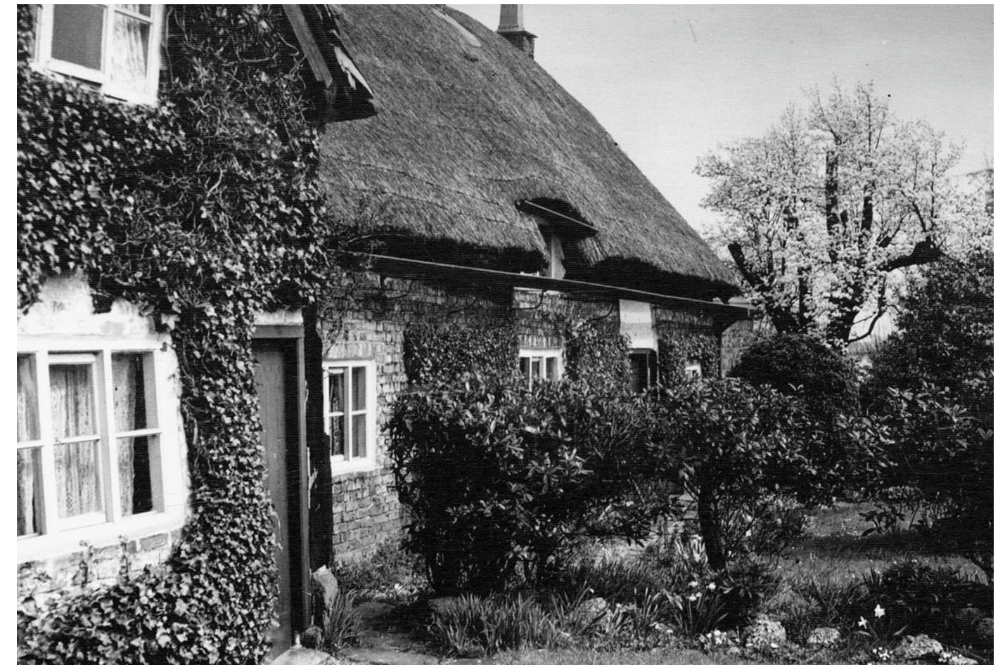
Figure 3: Photograph of Moss House Farm, Outwood Lane, in 1949. (Source: Image courtesy of Manchester Libraries, accession no. m49101).
