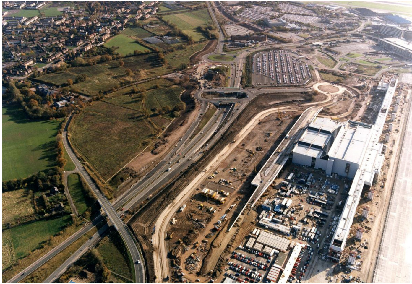
Figure 10: 1992 Photograph showing the improved road infrastructure works surrounding Manchester Airport. (Source: Image courtesy of Manchester Libraries, accession no. m83580).
