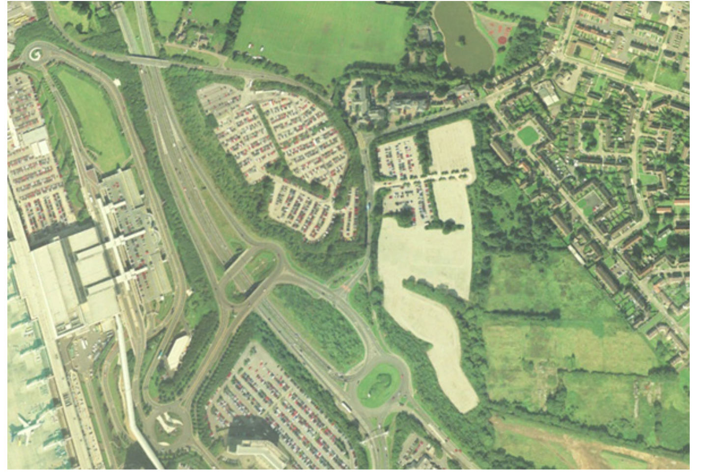
Figure 11: Aerial Image of the Site in December 2000 showing the new areas of car parking. (Source: Google Earth, December 2000).
