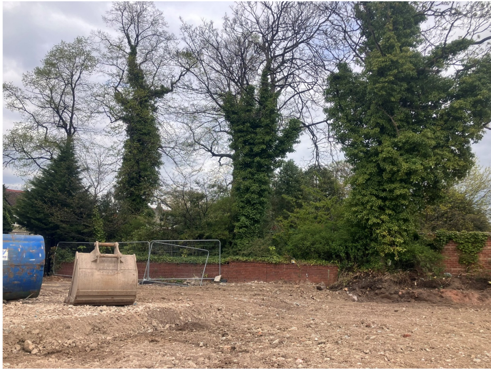
Photo P01A (Wall W01)
