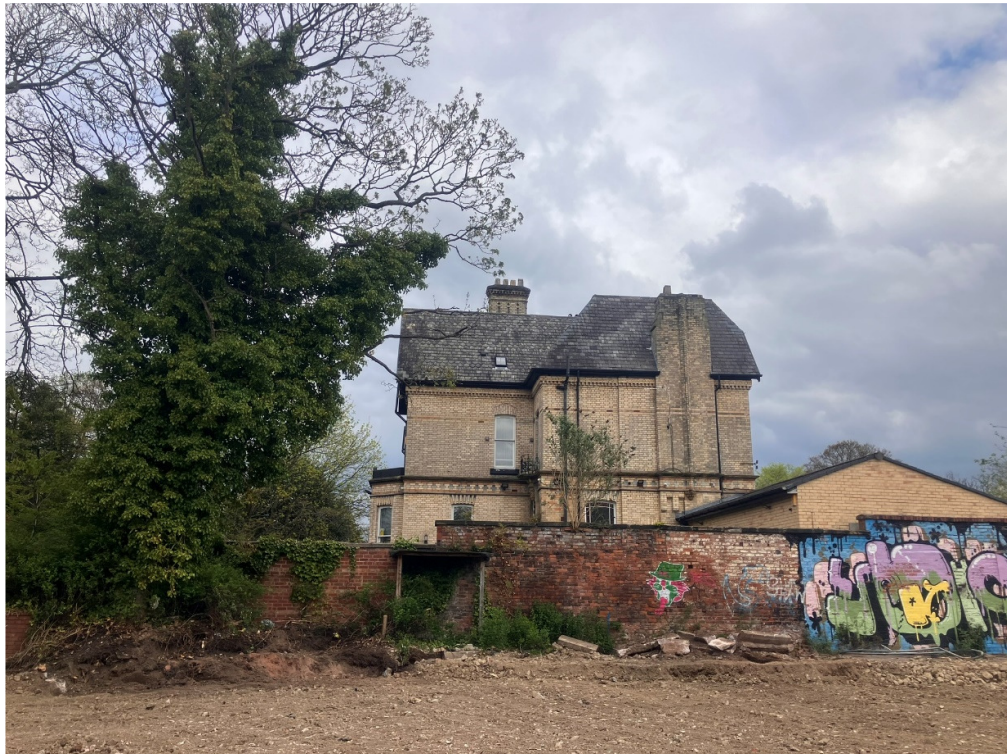
Photo P01B (Walls W01 & W02)
