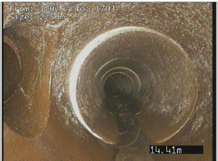
Junction at 9 o'clock, diameter 100mm
