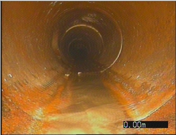
Start node type, manhole, reference 1702
