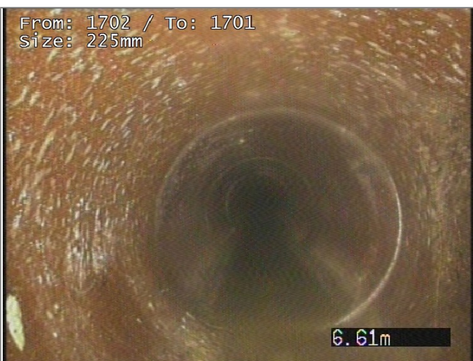
Junction at 3 o'clock, diameter 100mm
