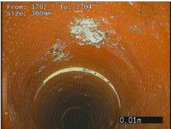
Junction at 9 o'clock, diameter 100mm
