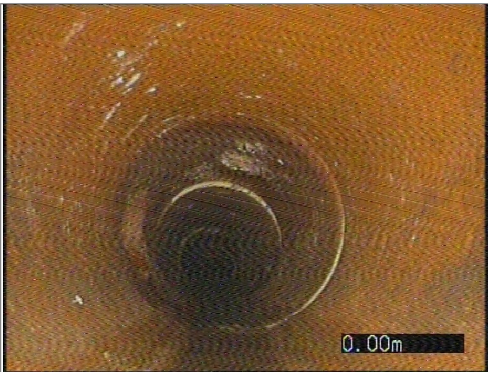
Start node type, manhole, reference 1702
