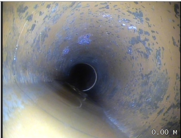
Start node type, manhole, reference 2602
