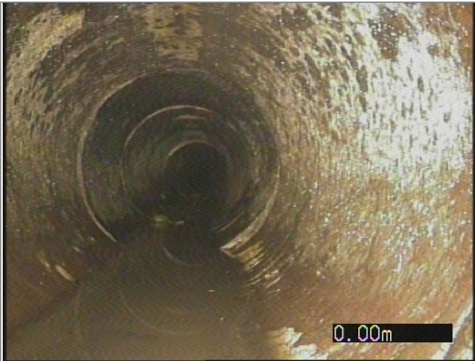
Start node type, manhole, reference 1703
