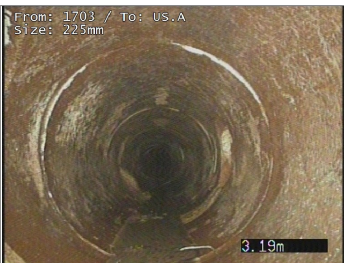
Junction at 9 o'clock, diameter 100mm
