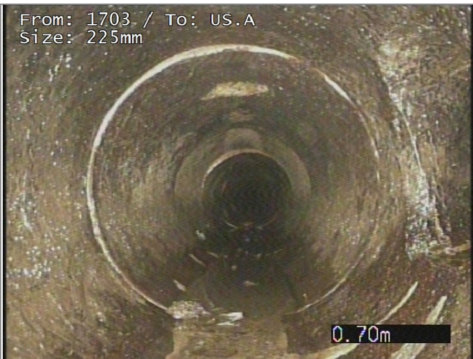
Junction at 3 o'clock, diameter 100mm
