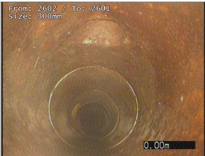
Junction at 12 o'clock, diameter 100mm
