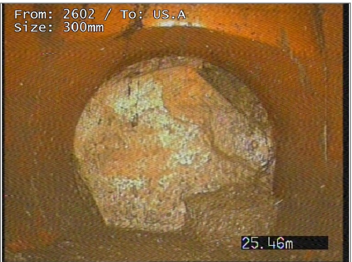
Junction at 12 o'clock, diameter 150mm
