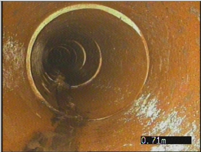
Start node type, manhole, reference 1702
