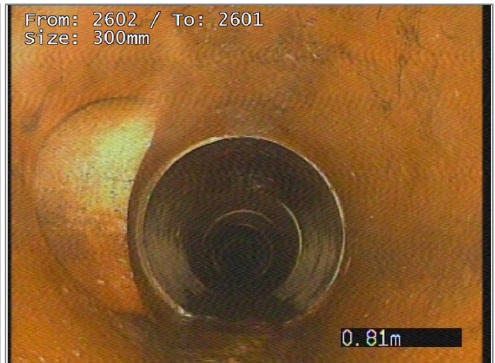
Junction at 9 o'clock, diameter 150mm
