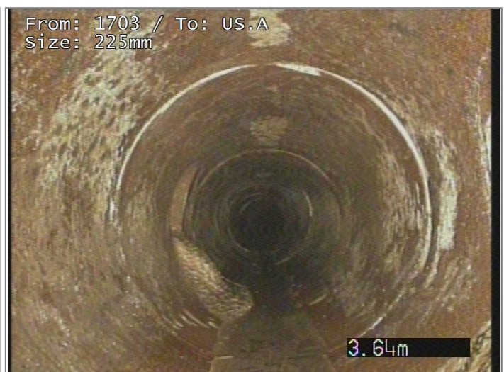
Junction at 3 o'clock, diameter 100mm
