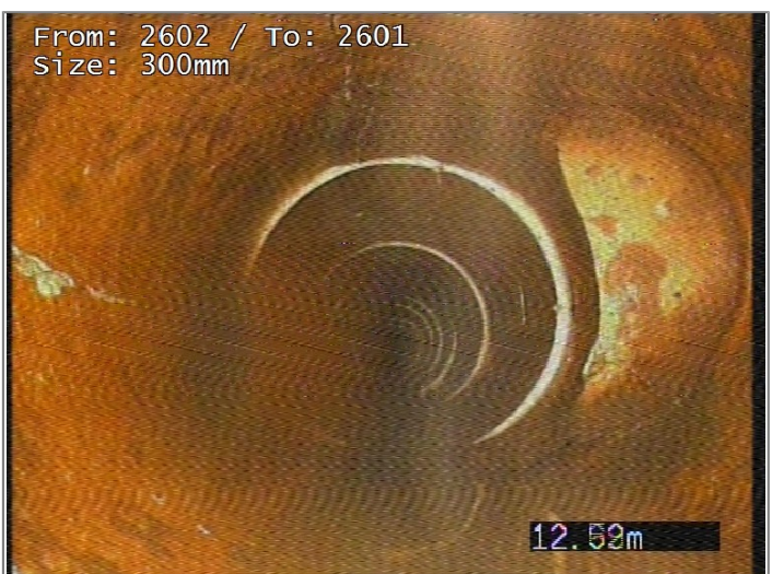
Junction at 3 o'clock, diameter 150mm
