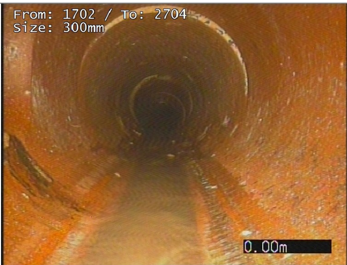
Junction at 9 o'clock, diameter 100mm
