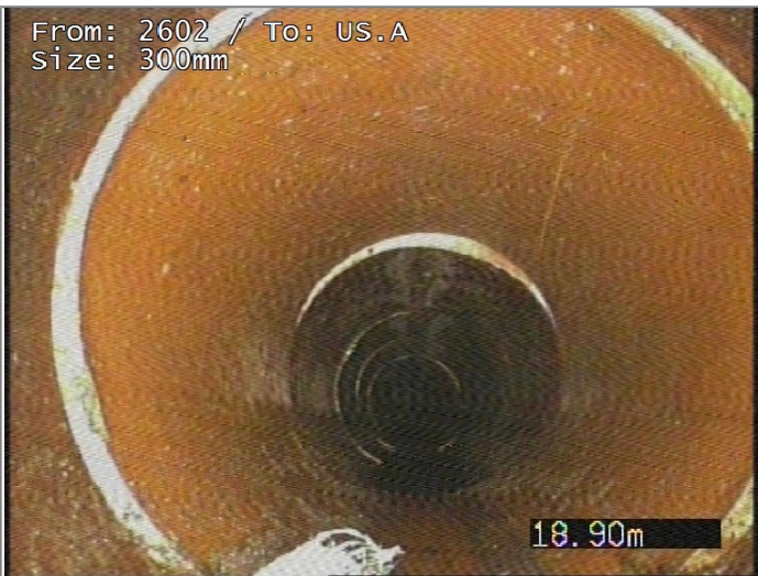
Junction at 3 o'clock, diameter 150mm
