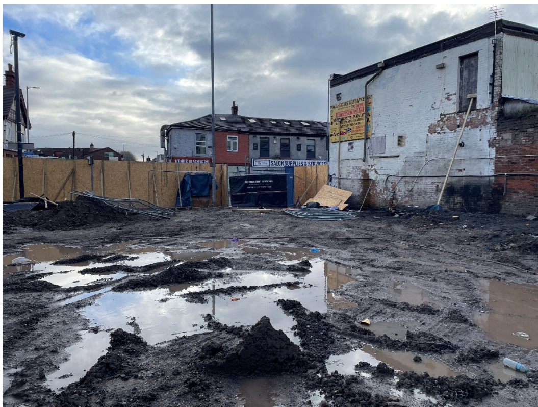
Photograph 11 - Site following demolition of existing structures
