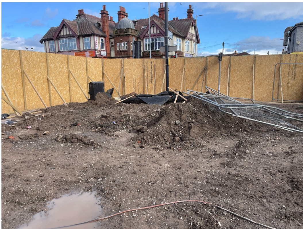
Photograph 13 - Site following demolition of existing structures
