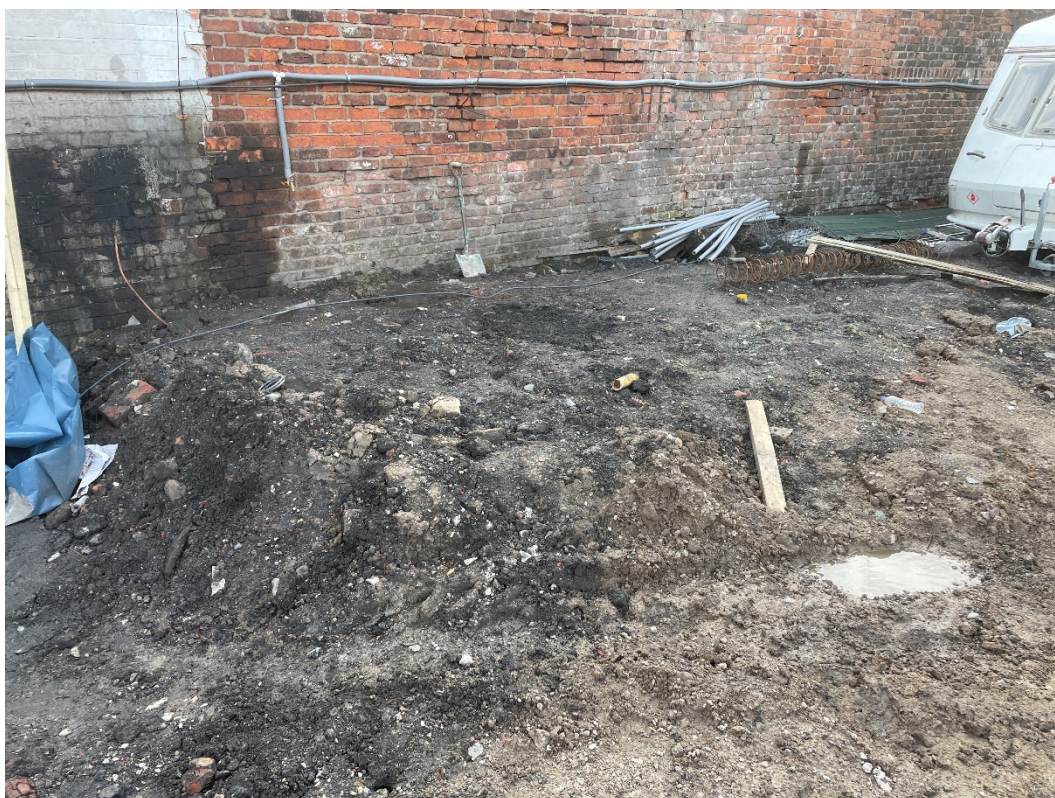
Photograph 12 - Site following demolition of existing structures
