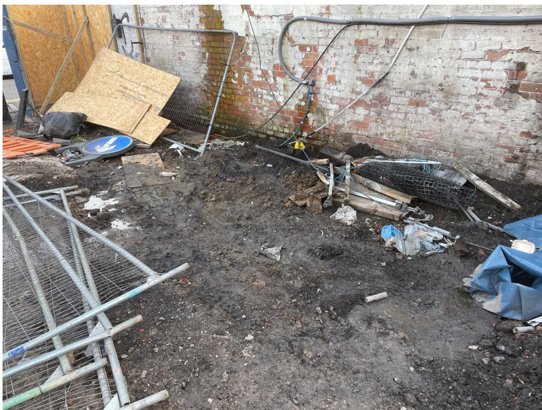
Photograph 14 - Site following demolition of existing structures
