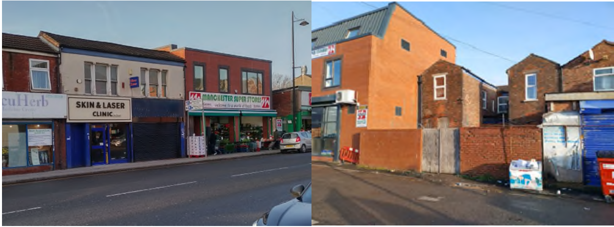
Fig.1 – Views of the front and rear of 50 Stockport Road
