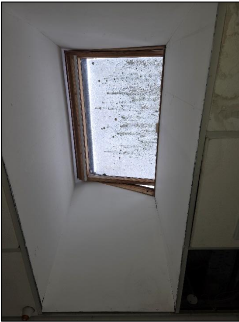
Photograph 21 showing partially open skylight
