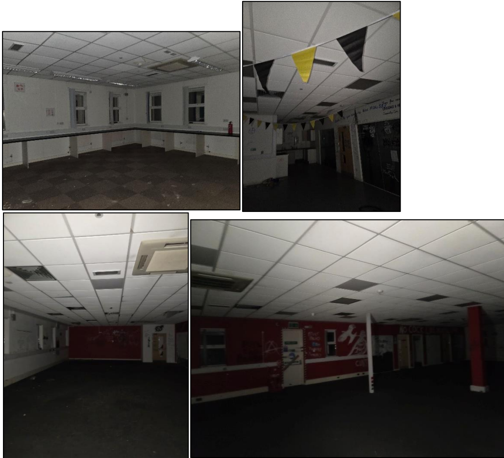
Photograph 17, 18, 19 & 20 showing the interior
