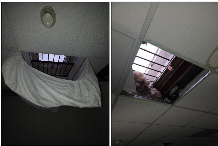
Photographs 22 & 23 showing the two vents present
