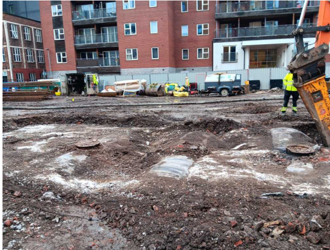
Photograph 1: View of 4no. tanks in situ before removal.
