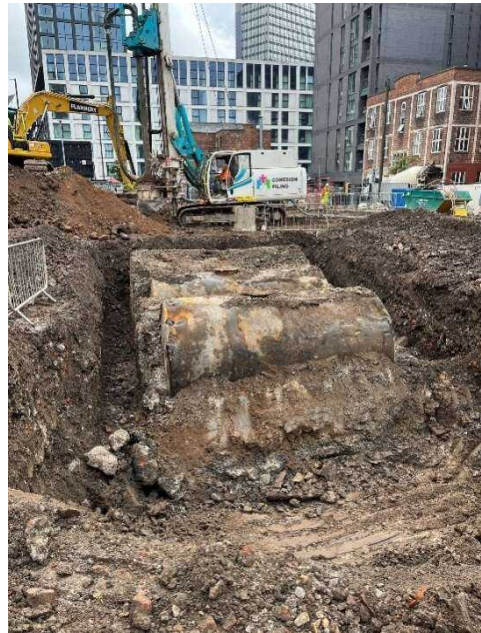
Photograph 2: View of exposed tanks and base of excavation of tank 1.
