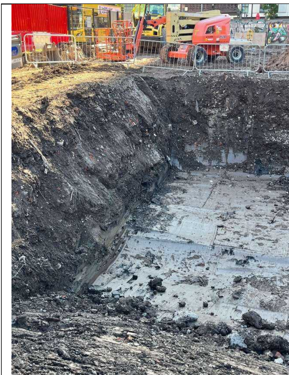
Photograph 3: View of southern side and base of pit after all tanks removed and material excavated.
