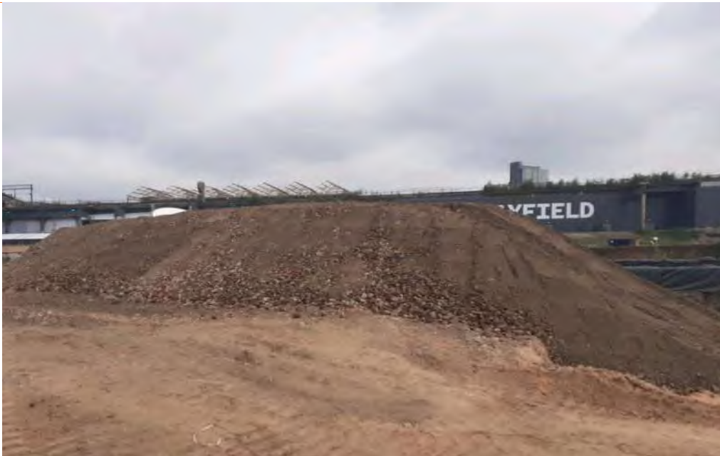
FIGURE 2 STOCKPILE OF ASHY MADE GROUND SAMPLED ON 8/6/21.
