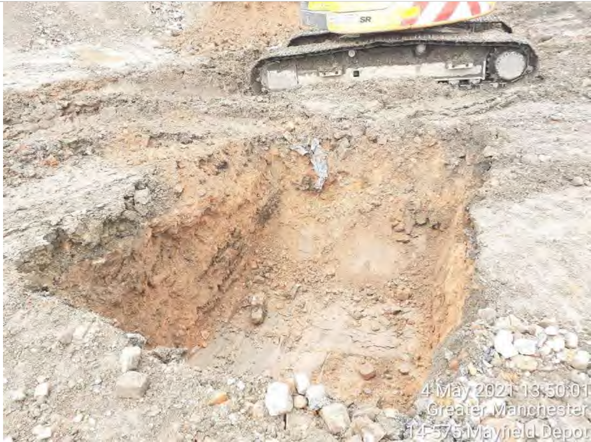
PLATE 7 TP103 HOTSPOT REMOVAL
