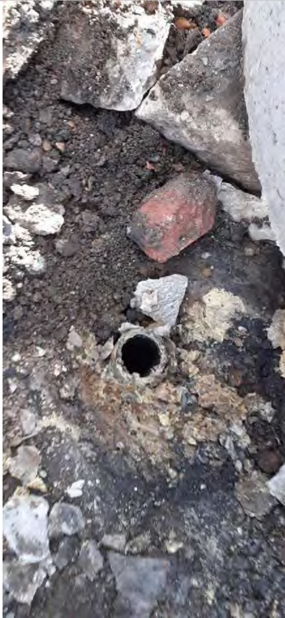
PLATE 12 GROUTING OF MONITOURING WELLS
