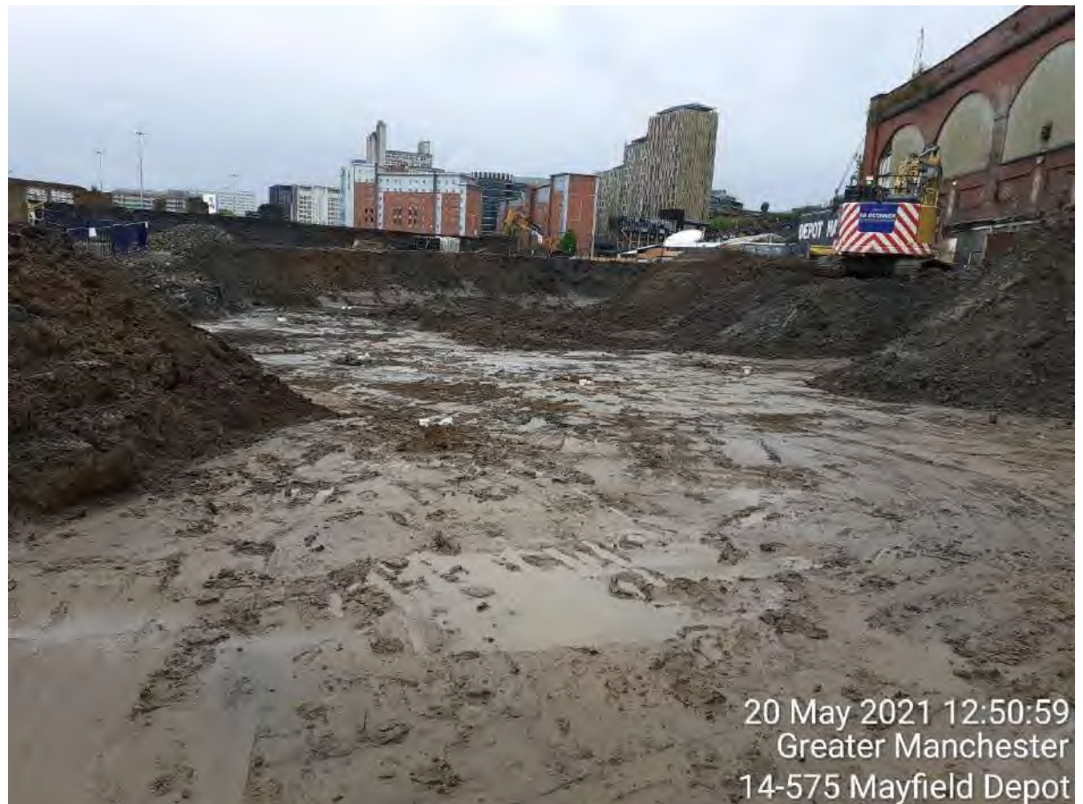
PLATE 9 HYDROCARBON SOURCE 1 REMOVAL
