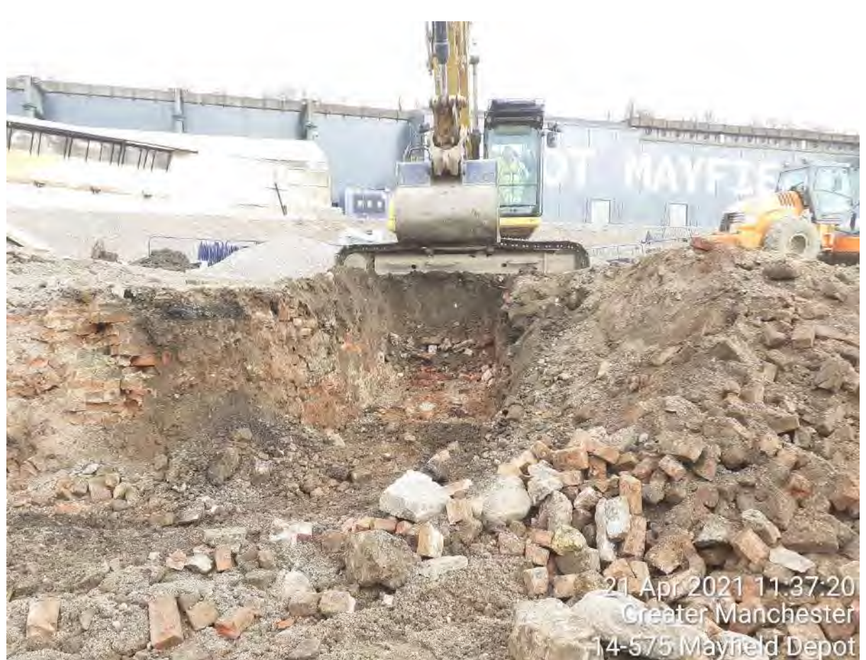
PLATE 10 HYDROCARBON SOURCE 3 HOTSPOT REMOVAL
