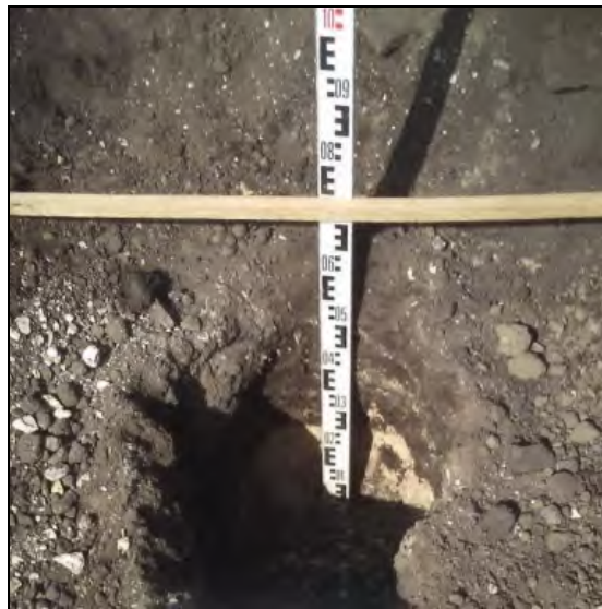
Fig 3.0 Example of soil capping depth validation photograph
