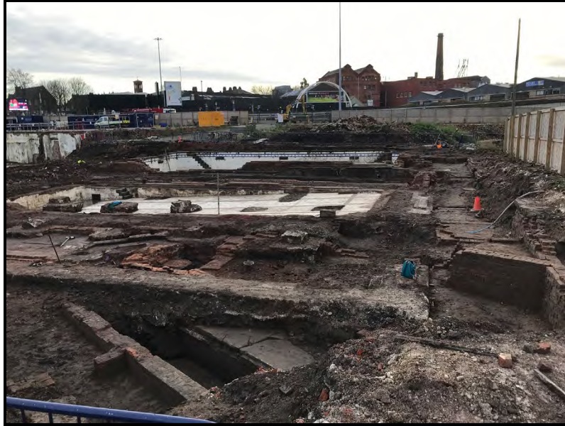
Plate 2.0: Mayfield Baths site following excavation
