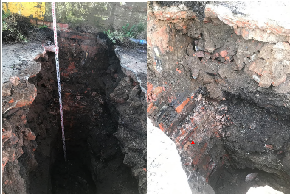
Stepped brick masonry
