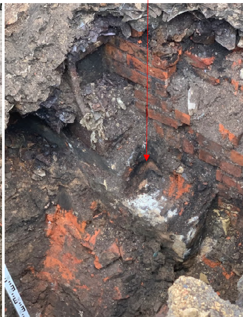
Hog's-back beam on padstone
