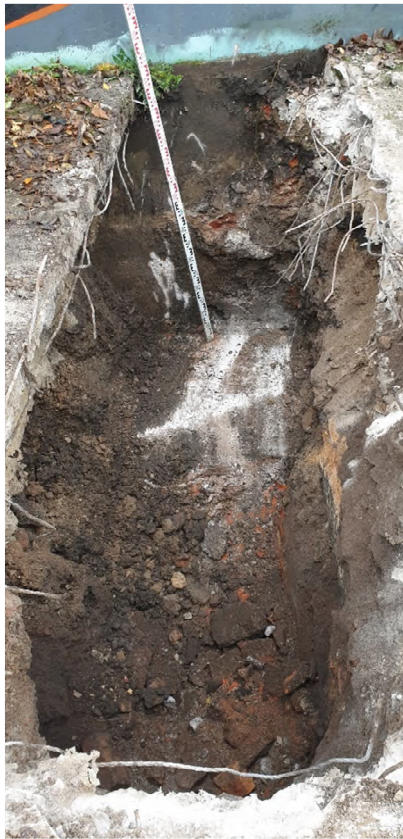
Plate No. 15: PP TPI09A – concrete footing at 1.6mbgl, extending out 1.0m and 1.0m deep
