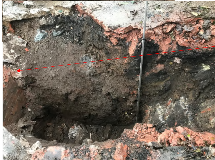
Parallel brick structure
