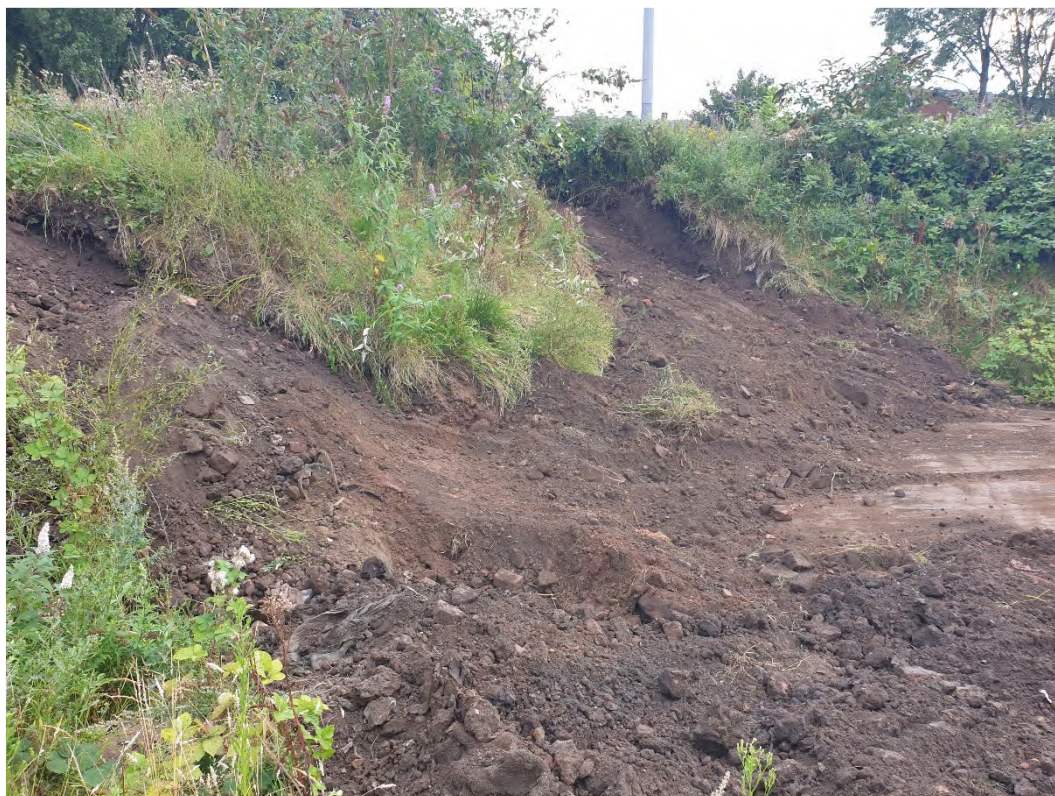
Photo No. 6: TP402 + TP402A locations
