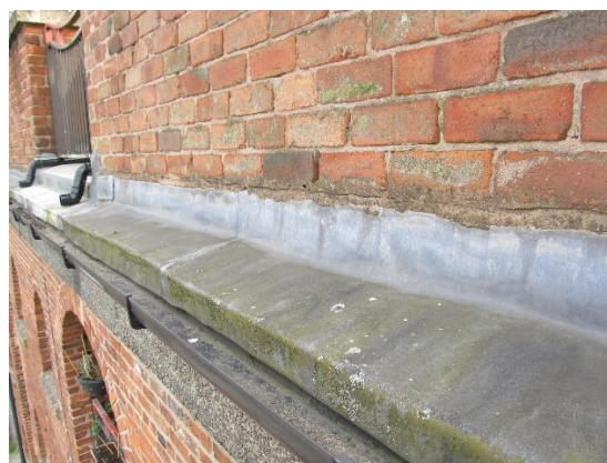
Leading edge to modern polymer polyethylene dpc / tray visible above the lead cover flashing.
