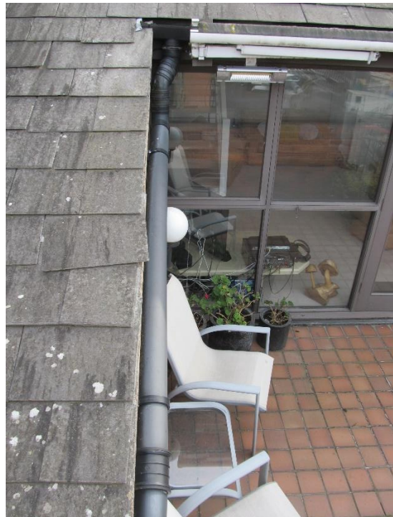
Drainage redirected from the eaves guttering to 503 roof terrace to the back gutter of 502.
