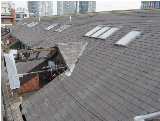
The rear roof slope drains to eaves guttering where cut-back to form the roof terraces.
