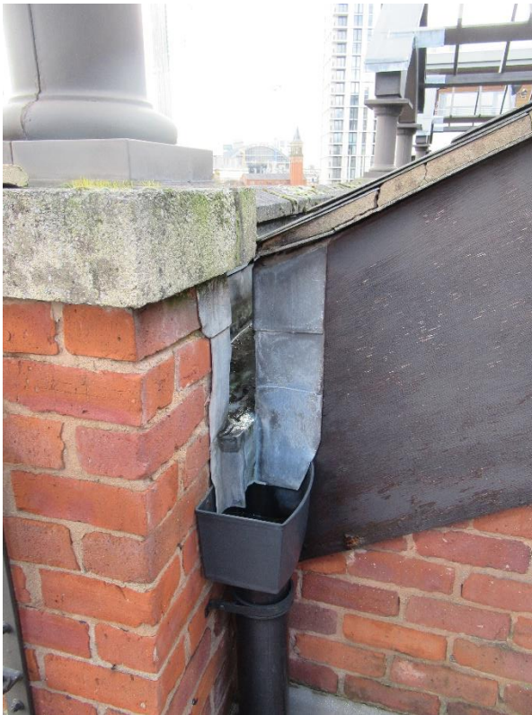
Hopper to open end of parapet gutter.
