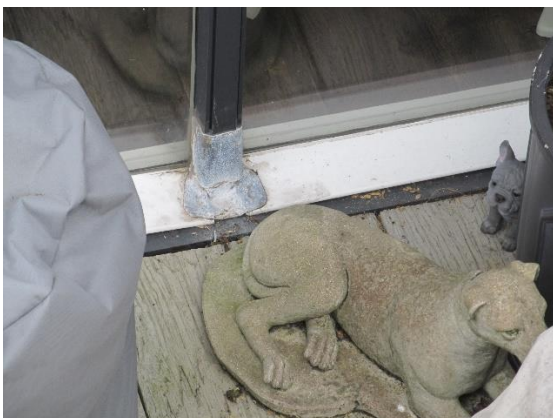
Further example of patch repairs to 504 Terrace.
