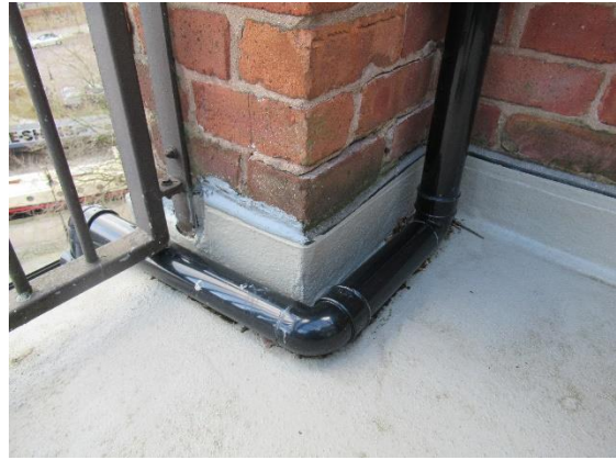
New liquid plastic overlay completed to a good standard and providing a watertight deck.
