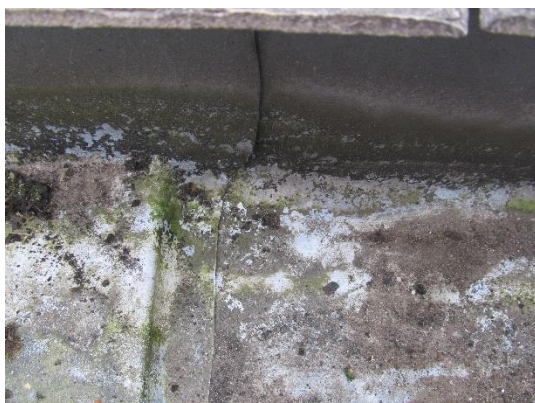
Standard joints to lengths of leadwork, sole and walls.
