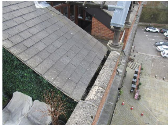
And to the hidden parapet gutters.
