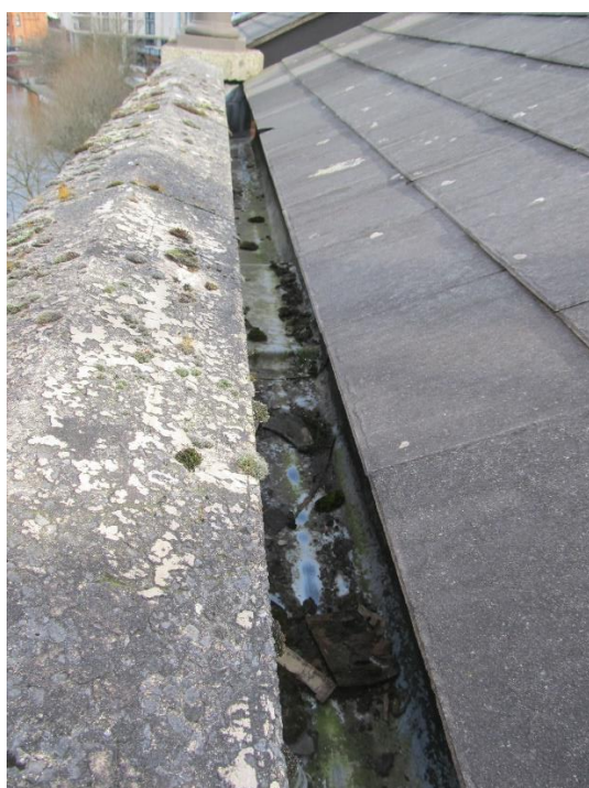
Given the length of the guttering the sections of lead have been jointed to prevent splitting.
