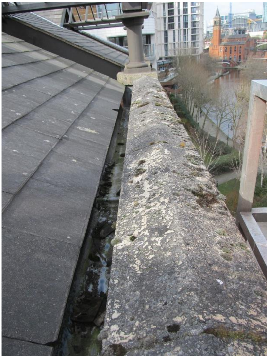
General arrangement of the back gutter.
