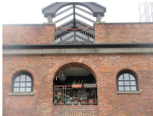
New build (1990s) construction above concrete ring beam.
