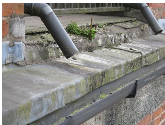
Downspouts serving the rear roof slopes and hidden parapet gutters.
