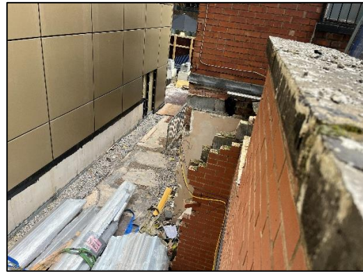
Plate 3. Large gap above the central window; partially demolished wall to the north.
