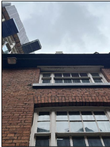
Plate 3. Large gap above the central window; partially demolished wall to the north.
