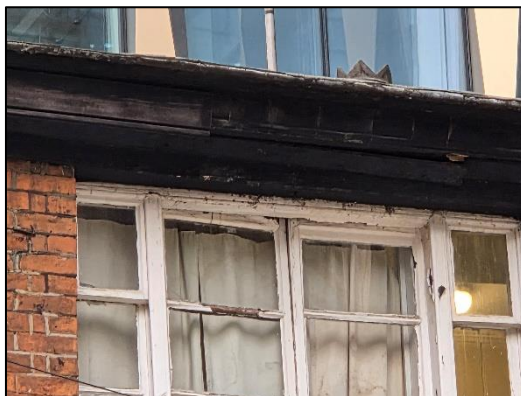
Plate 5: Gaps behind fascia boards.
