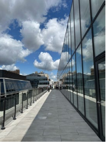
SITE PHOTOGRAPH (VIEWPOINT B)
