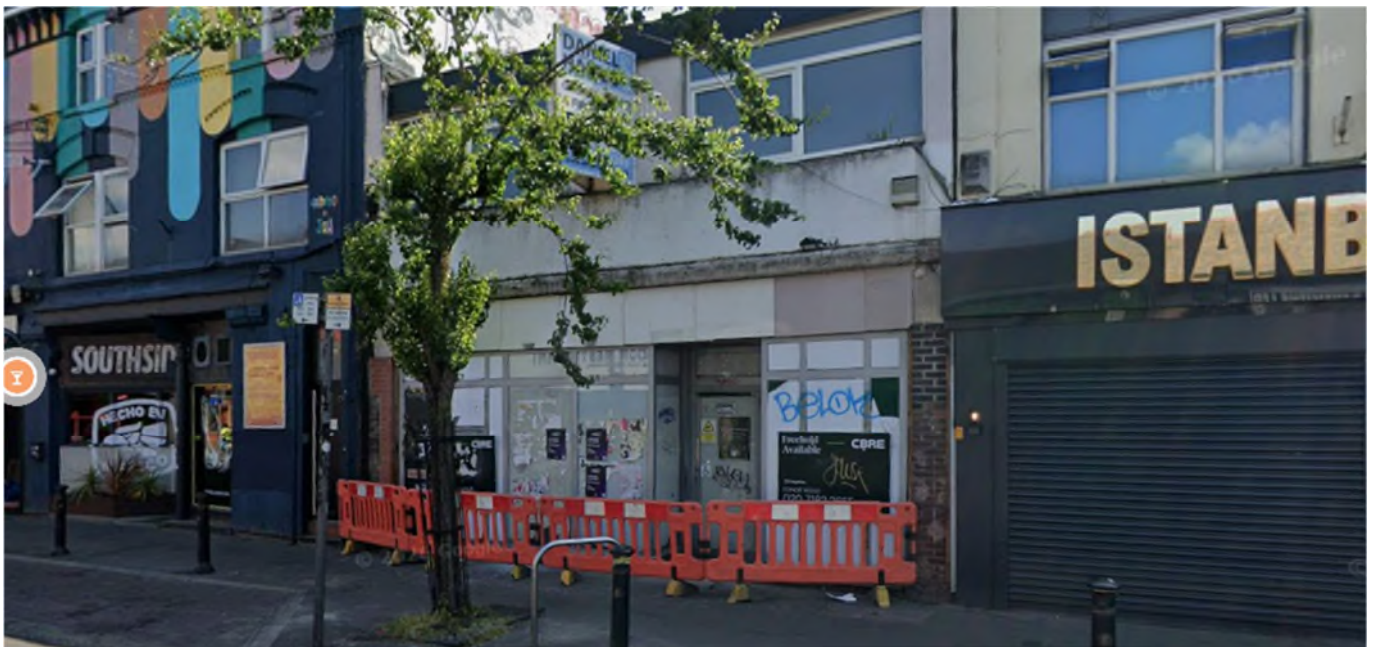
Application property in May 2025 prior to unauthorised works taking place
