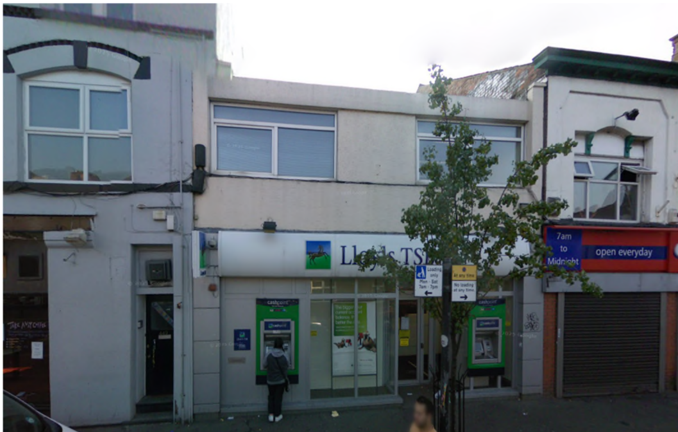
Application property in 2008 with render visible at first-floor level
