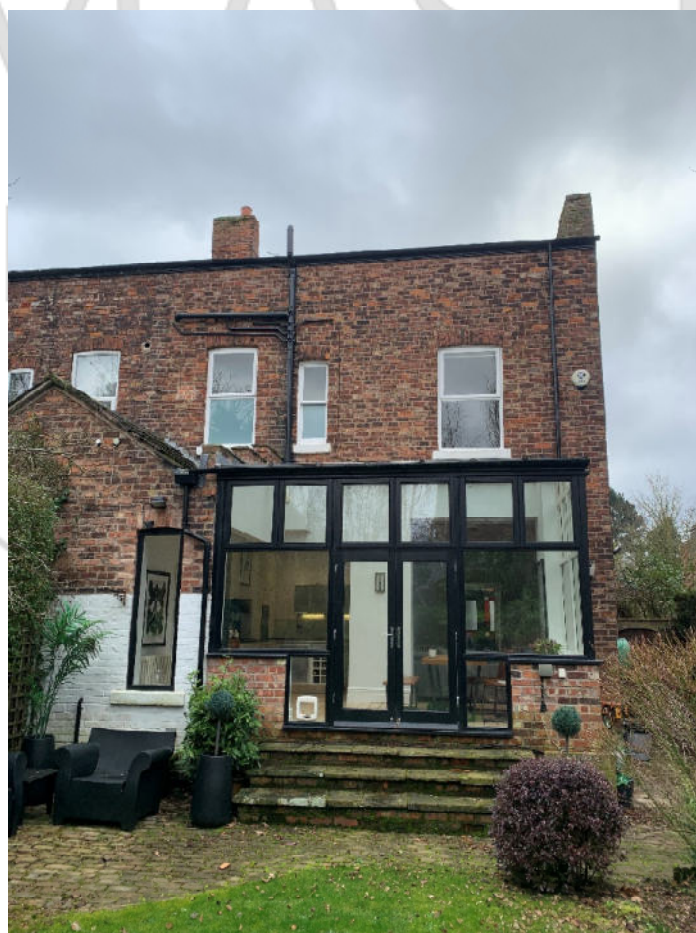
50 Old Lansdowne Road, Didsbury, Manchester – Rear Elevation
