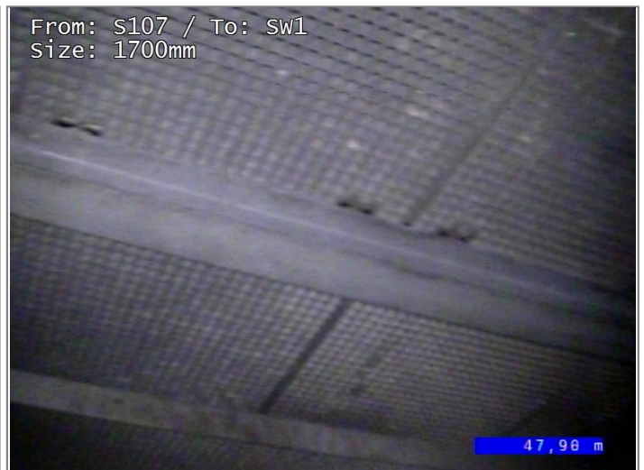
Finish node type, manhole, reference SW1
