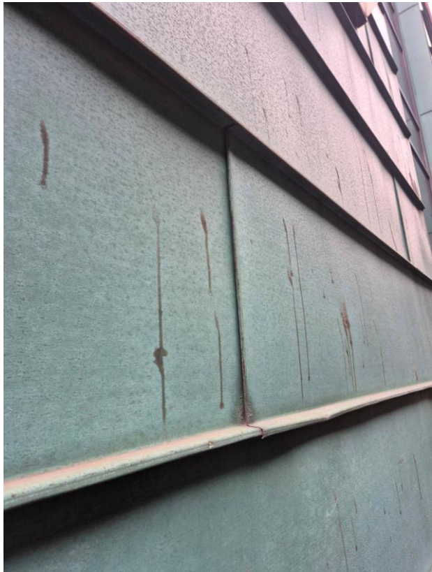
John Dalton HE Building Copper Cladding close-up
