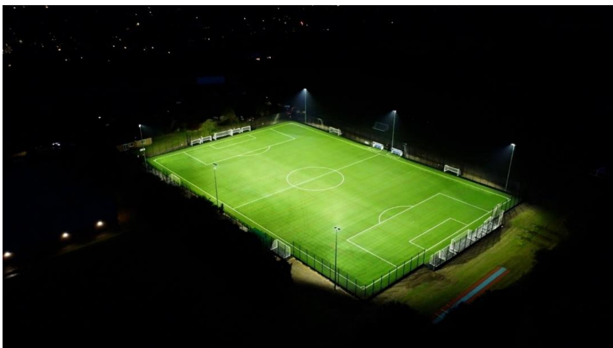
Figure 9 - Example AGP at Nighttime with Good LED Spill Control
