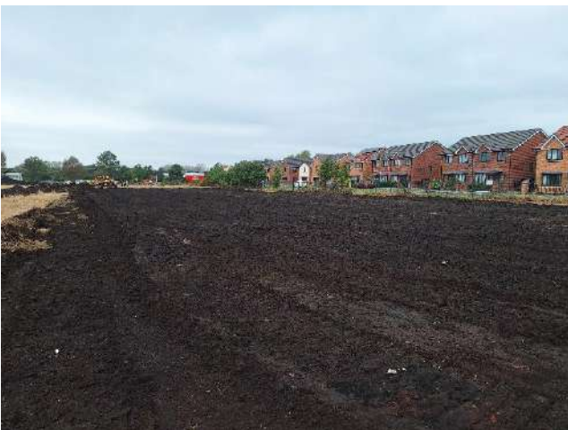
Photograph 5: North section prep for topsoil strip
