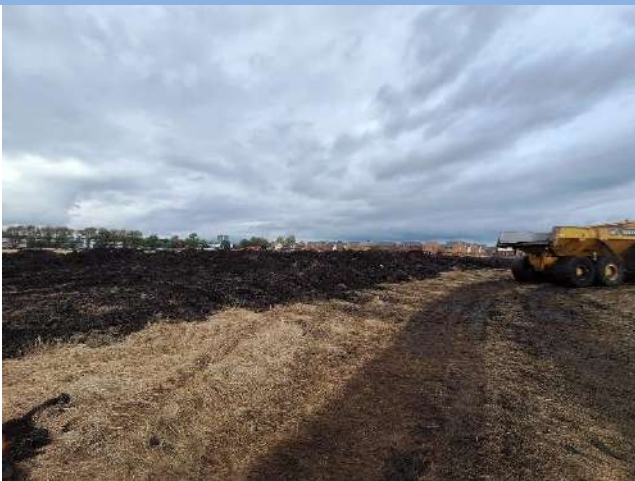
Photograph 11: Non-hazardous topsoil stockpile
