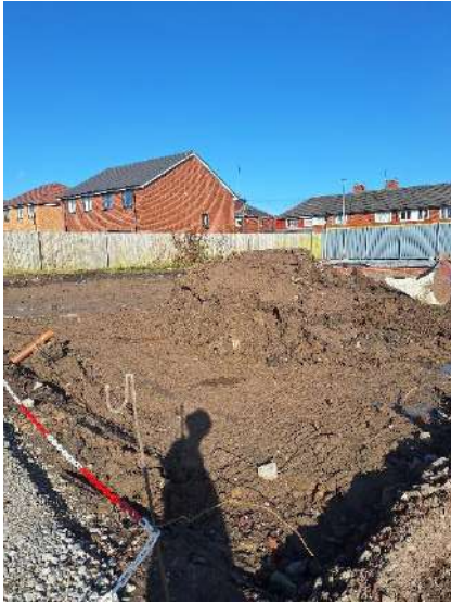
Photo 7: 24.02.25 – Stockpile 4 placed in plots
