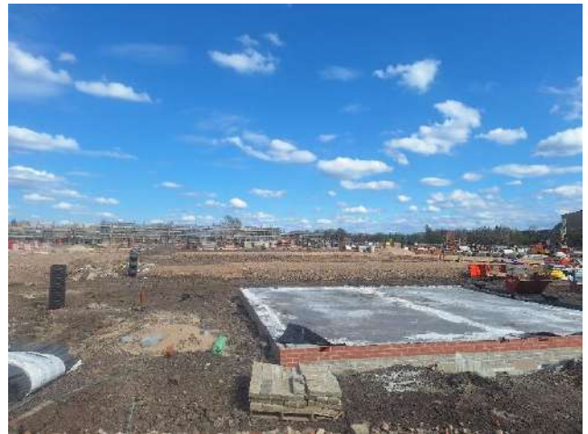
Photo 14: 17.04.25 – Site overview facing east
