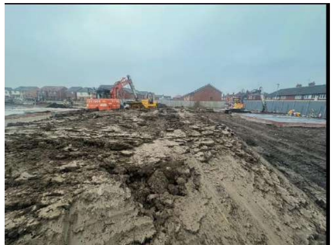
Photo 4: 18.02.25 – Made ground removed
