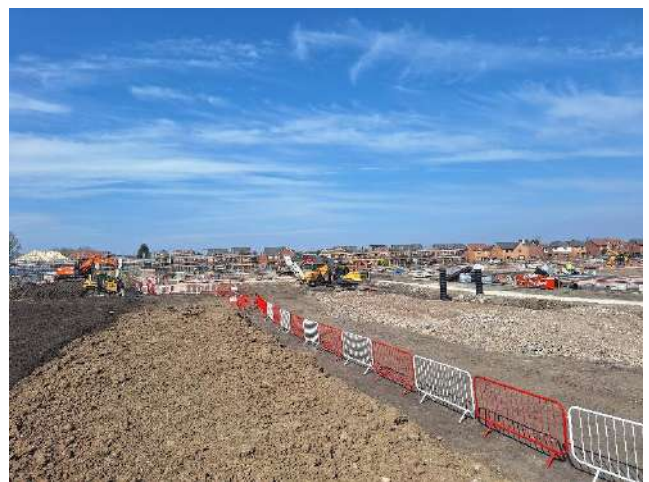
Photo 6: 03.04.25 – Site overview facing north
