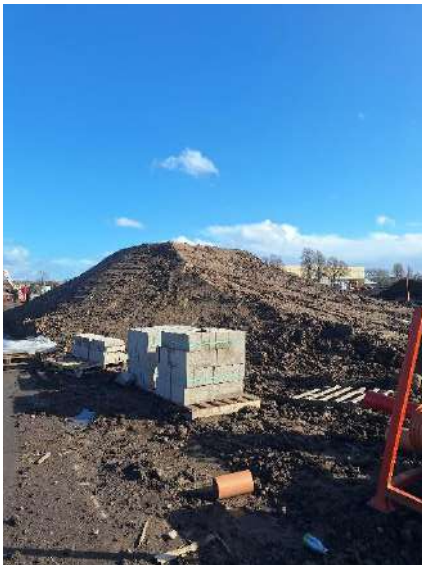
Photo 9: 24.02.25 – Subsoil stockpile from sewers
