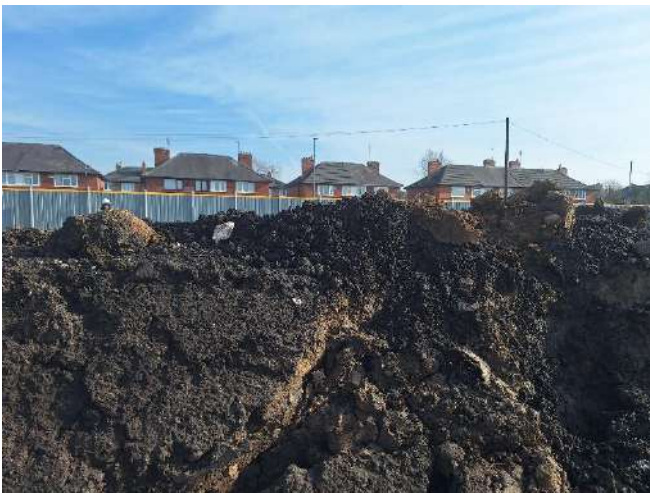
Photo 3: 18.02.25 – Stockpile 4 Made ground
