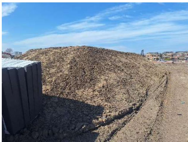
Photo 8: 03.04.25 – Stockpile 25 – Moved to centre of site
