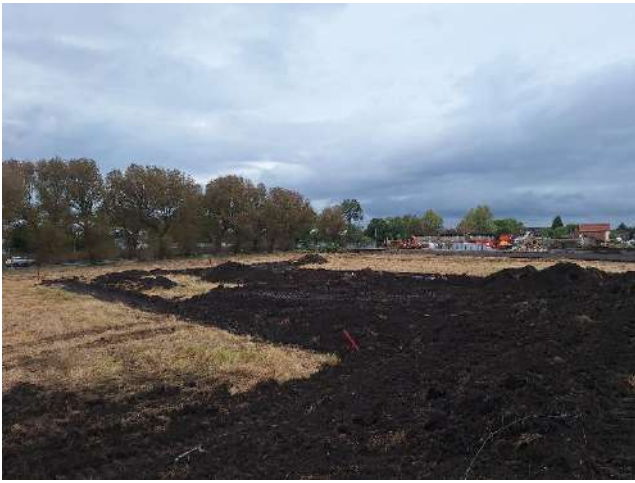
Photograph 9: TP186 area undergoing topsoil strip
