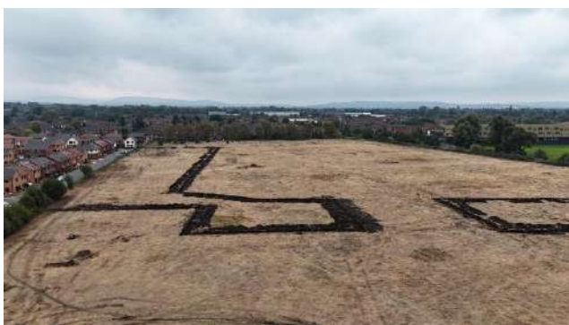
Photograph 1: Overview of hazardous topsoil areas
