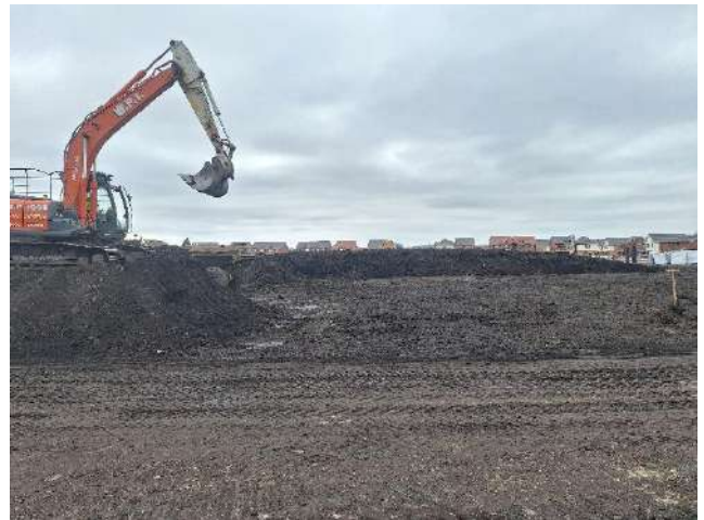
Photo 10: 03.03.25 – Non-hazardous topsoil export
