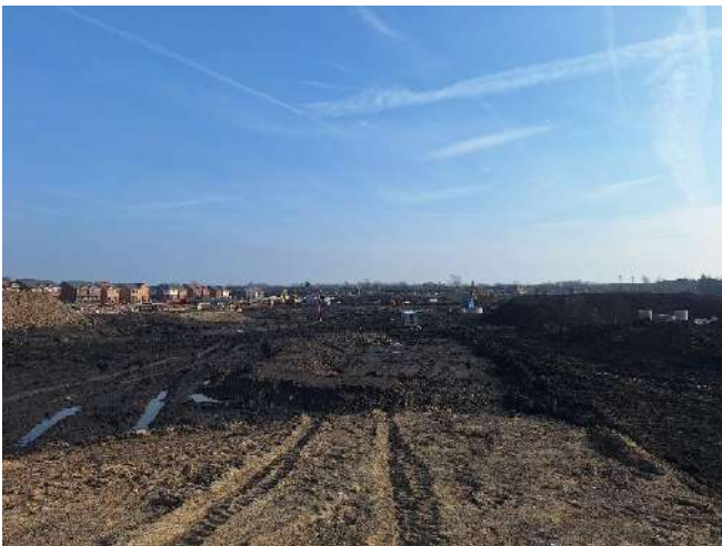
Photo 5: 18.02.25 – Site overview facing east
