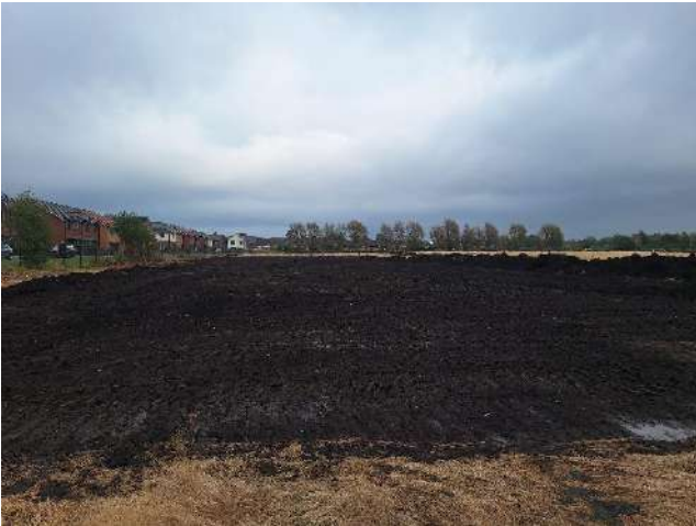
Photograph 3: North section prep for topsoil strip
