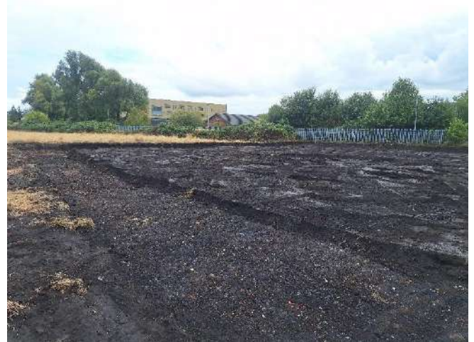
Photograph 10: TP219 topsoil strip complete
