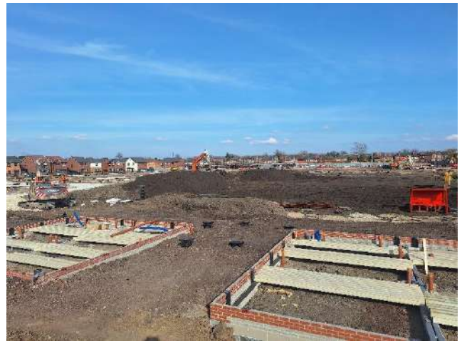
Photo 14: 20.03.25 – Remaining non-hazardous topsoil for export
