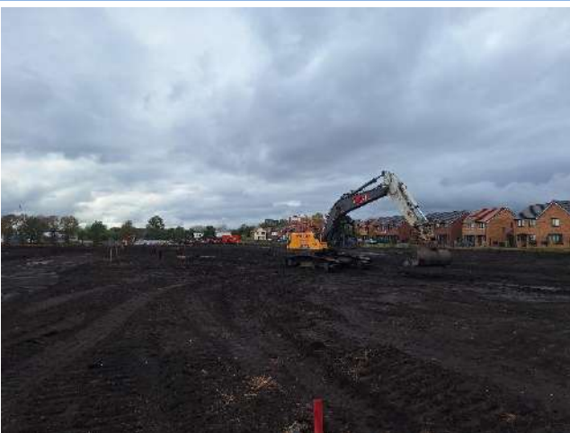
Photograph 7: North section following topsoil removal
