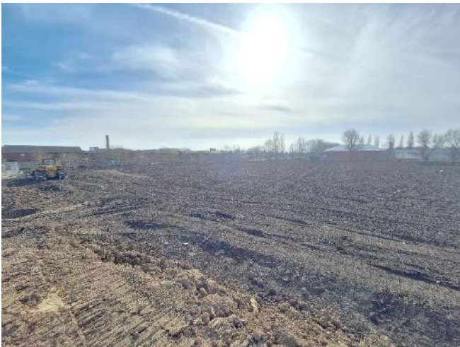
Photo 16: 20.03.25 – Hazardous topsoil placement
