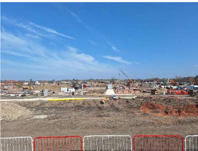
Photo 5: 03.04.25 – Site overview facing east
