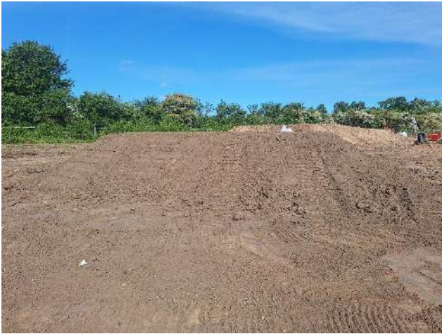
Photograph 1 – Stockpile facing north
