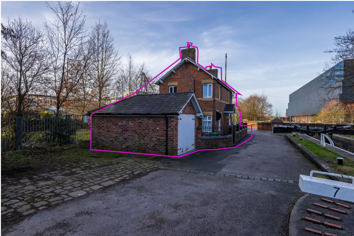
Figure 20 Ashton Canal Lock Keepers Cottage on South Side of Lock Number 7 of Ashton Canal (Source: Planit, February 2026) Asset outlined in pink
