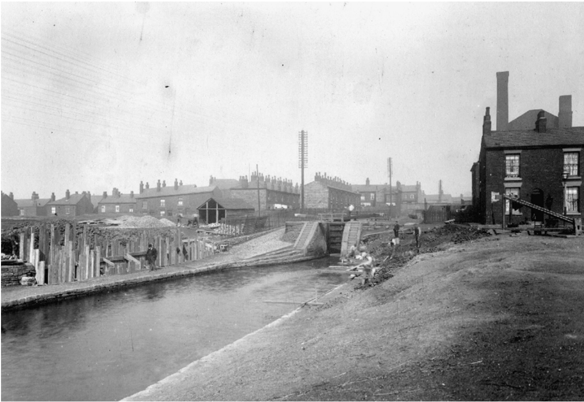
Figure 5: Forge Lane site for bridge over Canal (A Bradburn, 1903). Photo taken looking north east, with Canal Lock 6 visible at the centre of the image. The Site is located to the right side of the canal, Bradford Mill can be seen in the background to the right side of the frame.
