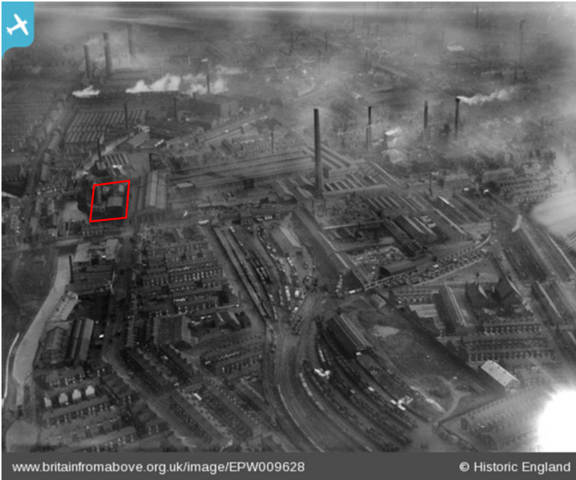
Figure 9: The Bradford Iron Works, Manchester, 1923 (Source: Britain from Above). Site just visible to the left the image, indicated in red
