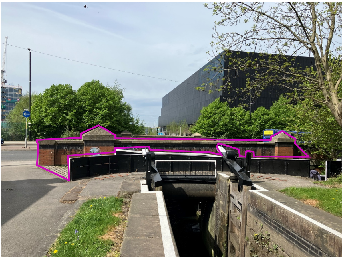
Figure 21 Mill Bridge (Source: Authors own, April 2025) Asset outlined in pink.
