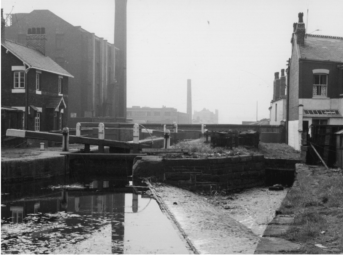
Figure 11 Ashton-under-Lyne Canal: 141, Manchester, Mill Street Bridge (L Kaye, 1960). Looking west toward Mill Street Bridge, with Lock Keepers cottage to left side of frame, and Lock 7 in the foreground. The Site is located in background, to the left beyond Mill Street bridge.
