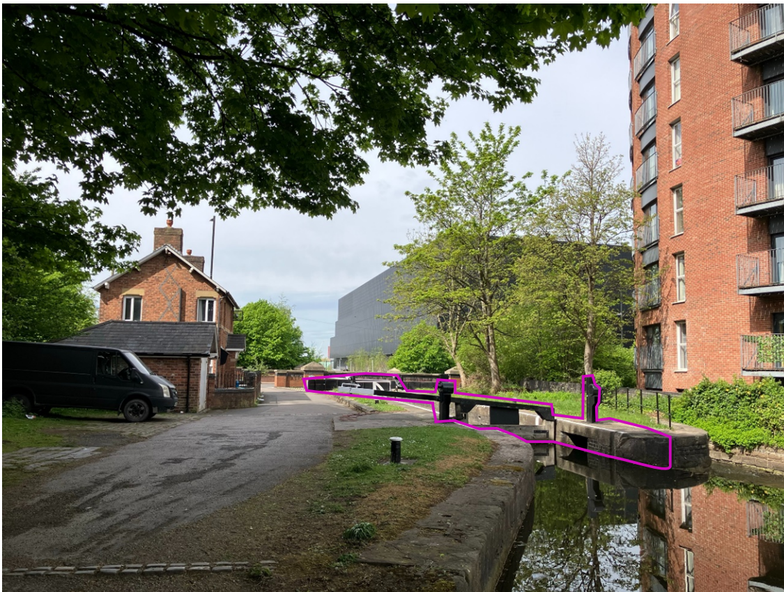
Figure 19 Ashton Canal Lock Number 7 with Roving Bridge Immediately East of Mill Street Bridge (Source, Authors Own, April 2025) Asset outlined in pink
