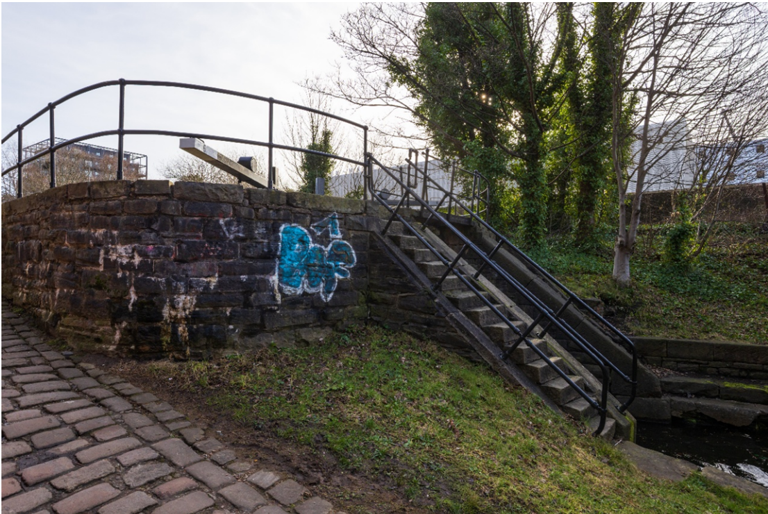
Figure 24 Looking south-east along Ashton Canal (Source: Planit, 2026). Proposed development shown as rendered
