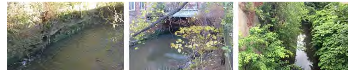
Figure 4-1 Existing river walls
