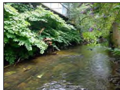
Looking upstream showing overhanging structure on right bank
