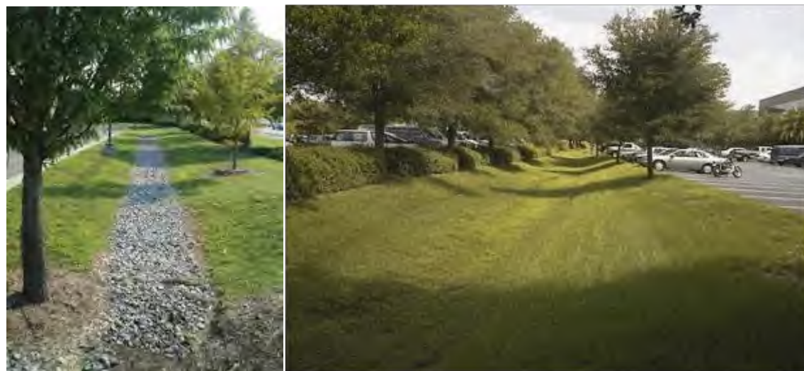
Figure 7-2 Infiltration Trench Example (Left); Swale Example (Right)
