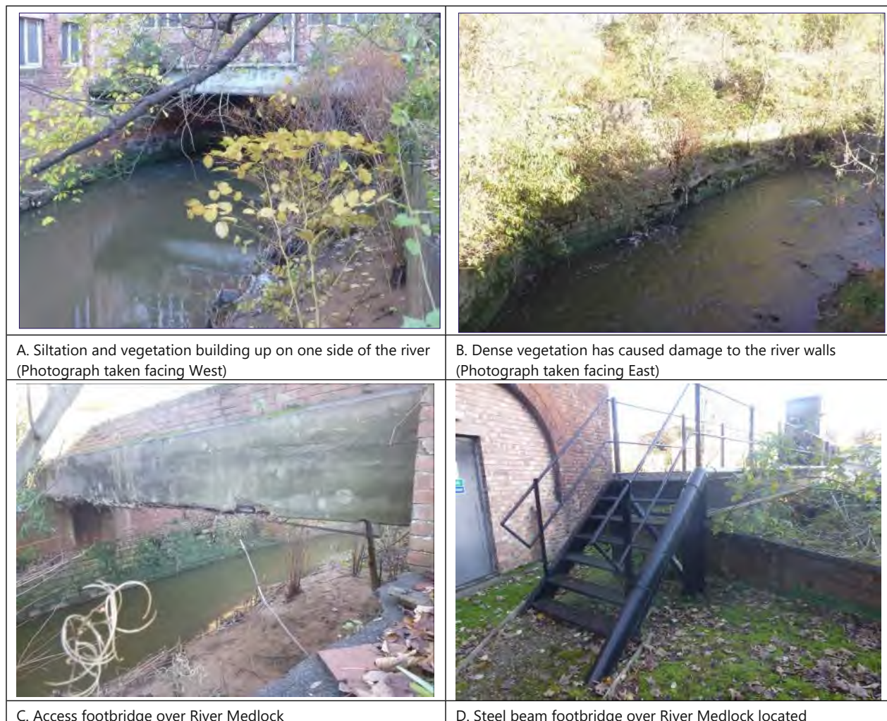
Figure 4.1 - Photos from past site visits
