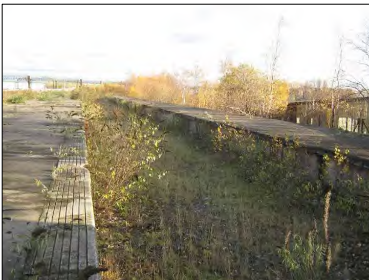
Plate 3 - Vegetated former railway tracks, looking towards dense birch woodland
