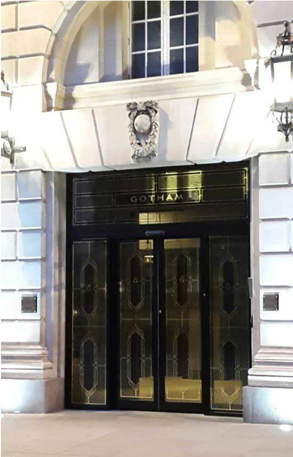
Existing Entrance Treatment
