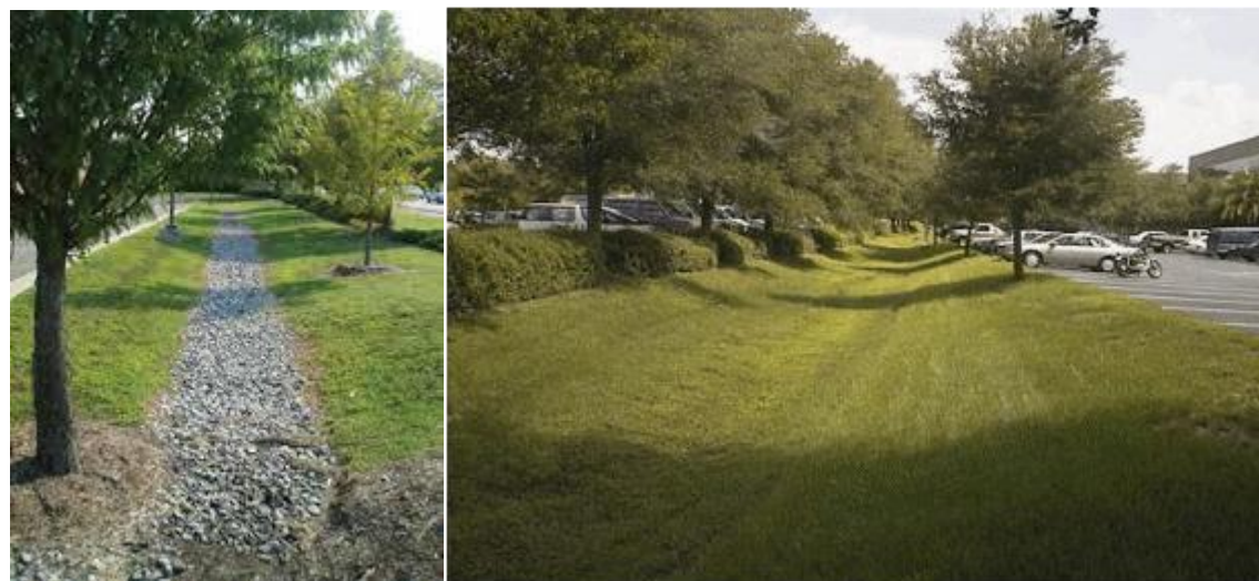
Figure 7-2 Infiltration Trench Example (Left); Swale Example (Right)
