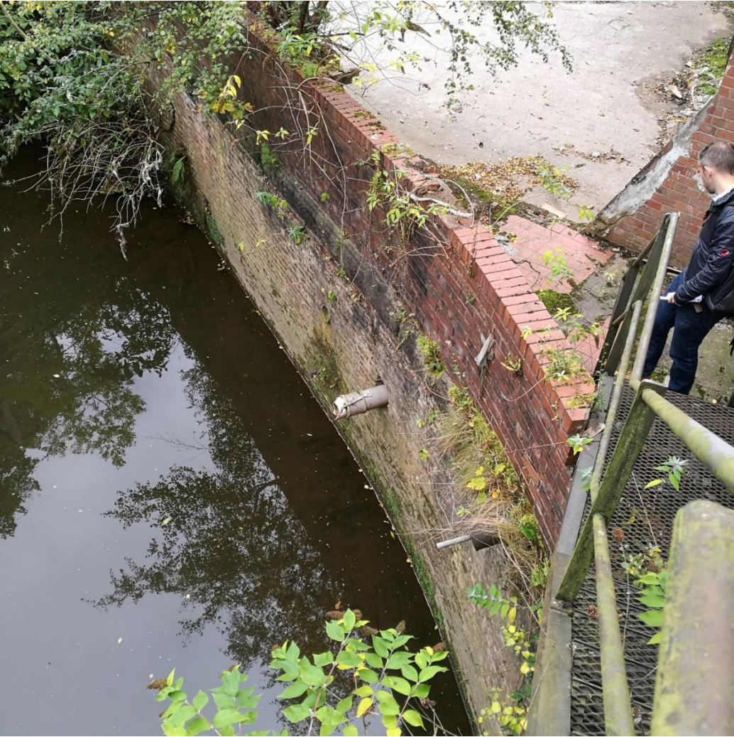
Figure 5-1 Existing Outfall Observed During Site Visit
