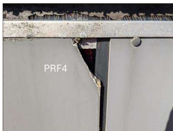
Photograph 6. PRF4 closely inspected by MEWP.
