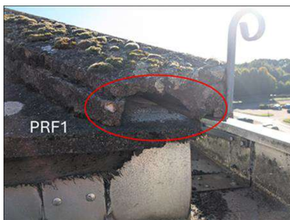
Photograph 3. PRF1 closely inspected by MEWP.
