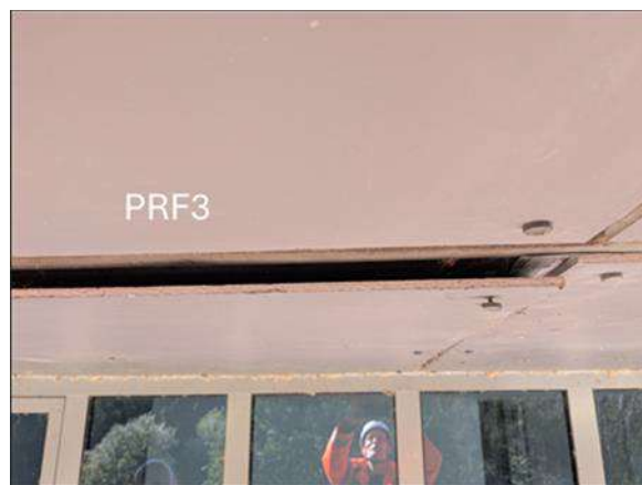
Photograph 5. PRF3 closely inspected by MEWP.
