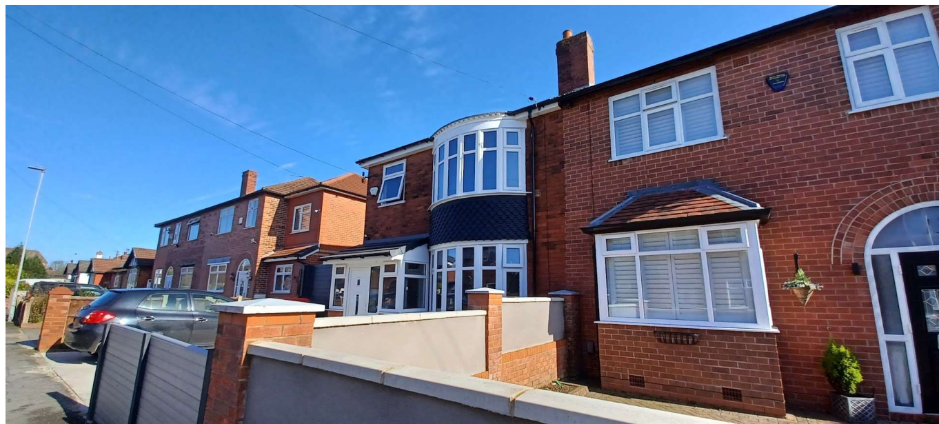
Two-storey front bay evident at No.11 Omer Drive
