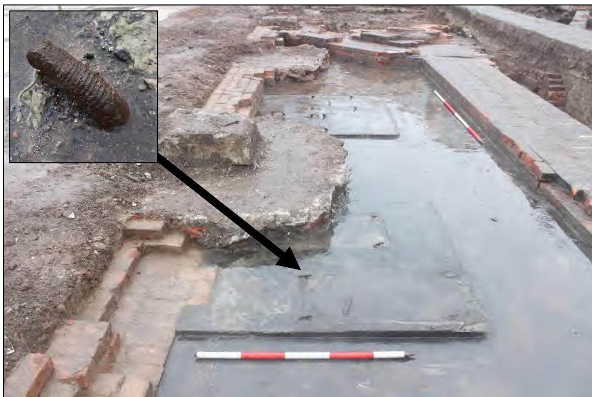
Plate 66: Anteroom to the boiler showing stone machine beds 216a (foreground) and 216b in the rear of the shot (1m and 2m scales) Inset: showing threaded bolt
