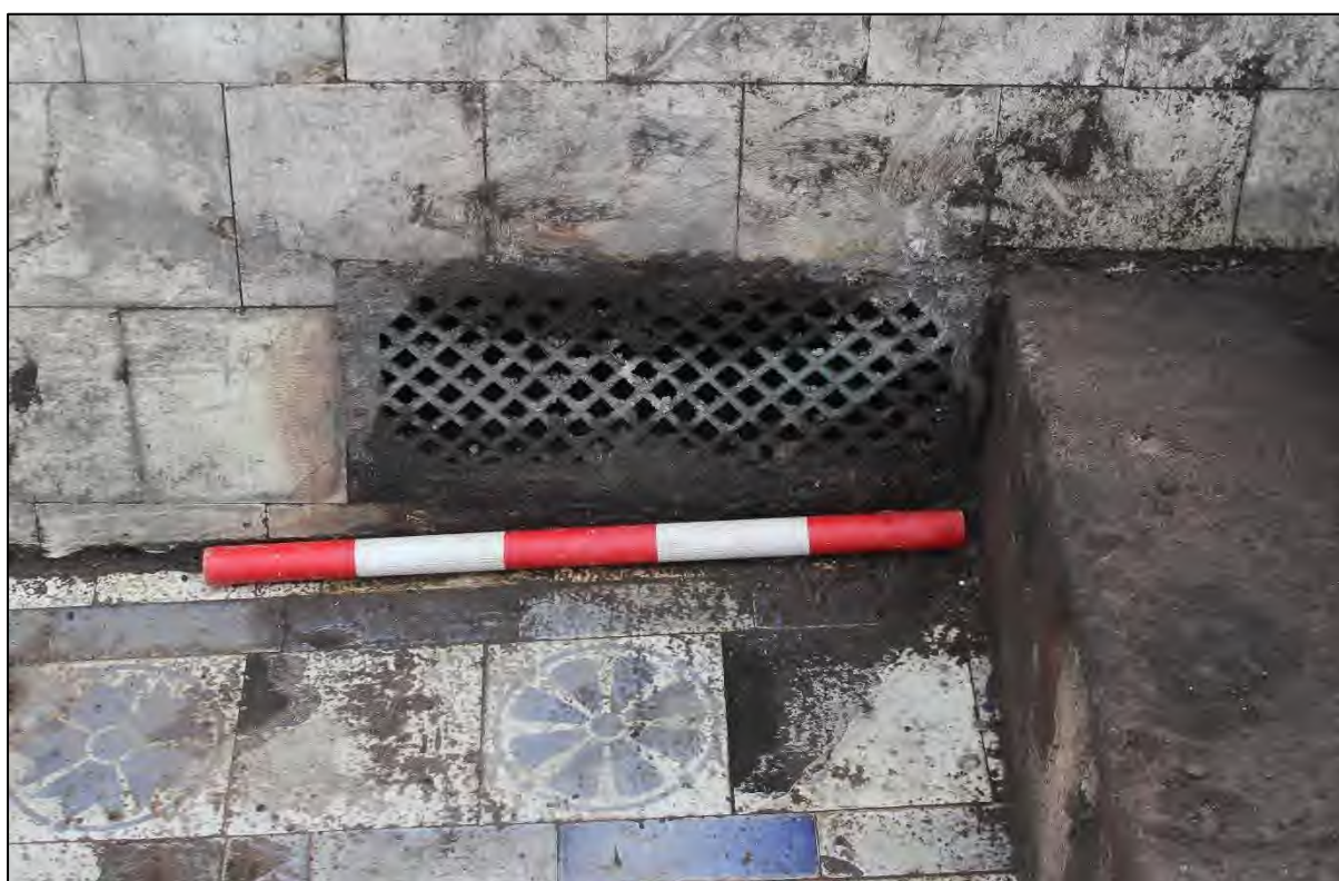
Plate 65: Brass grate at the south-west corner of Pool 225 (0.50m scale)
