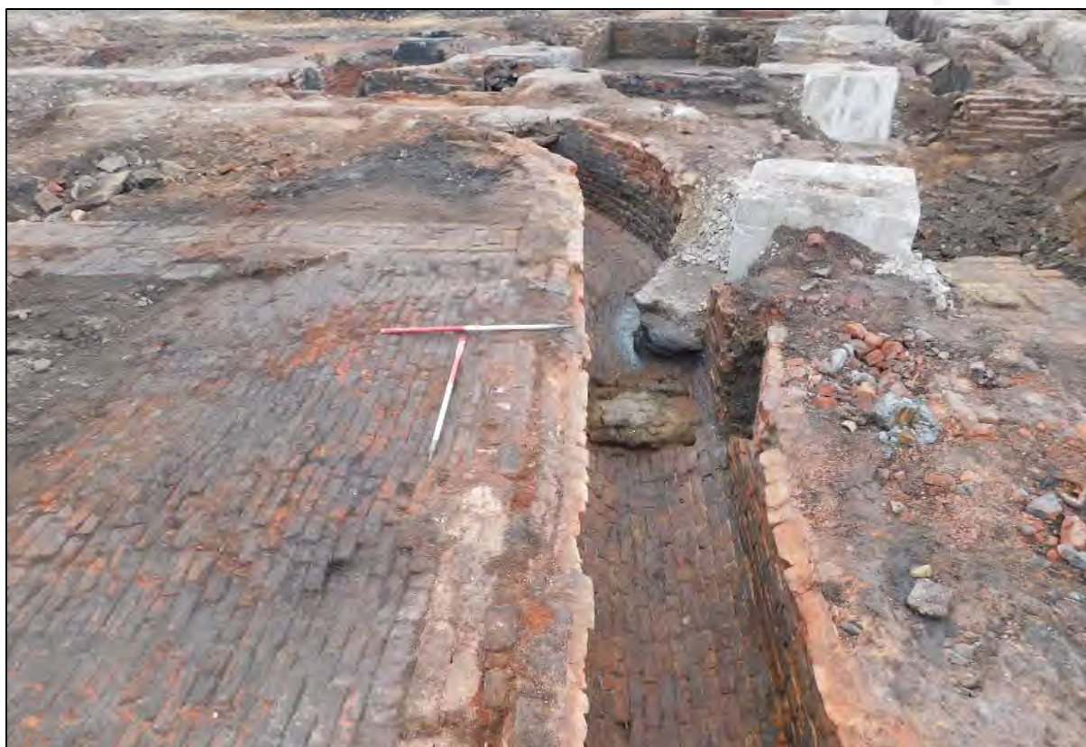
Plate 166: Flue 425 cutting surface 405 and wall 406 with modern concrete truncation, facing south east (2 x 1m scales)
