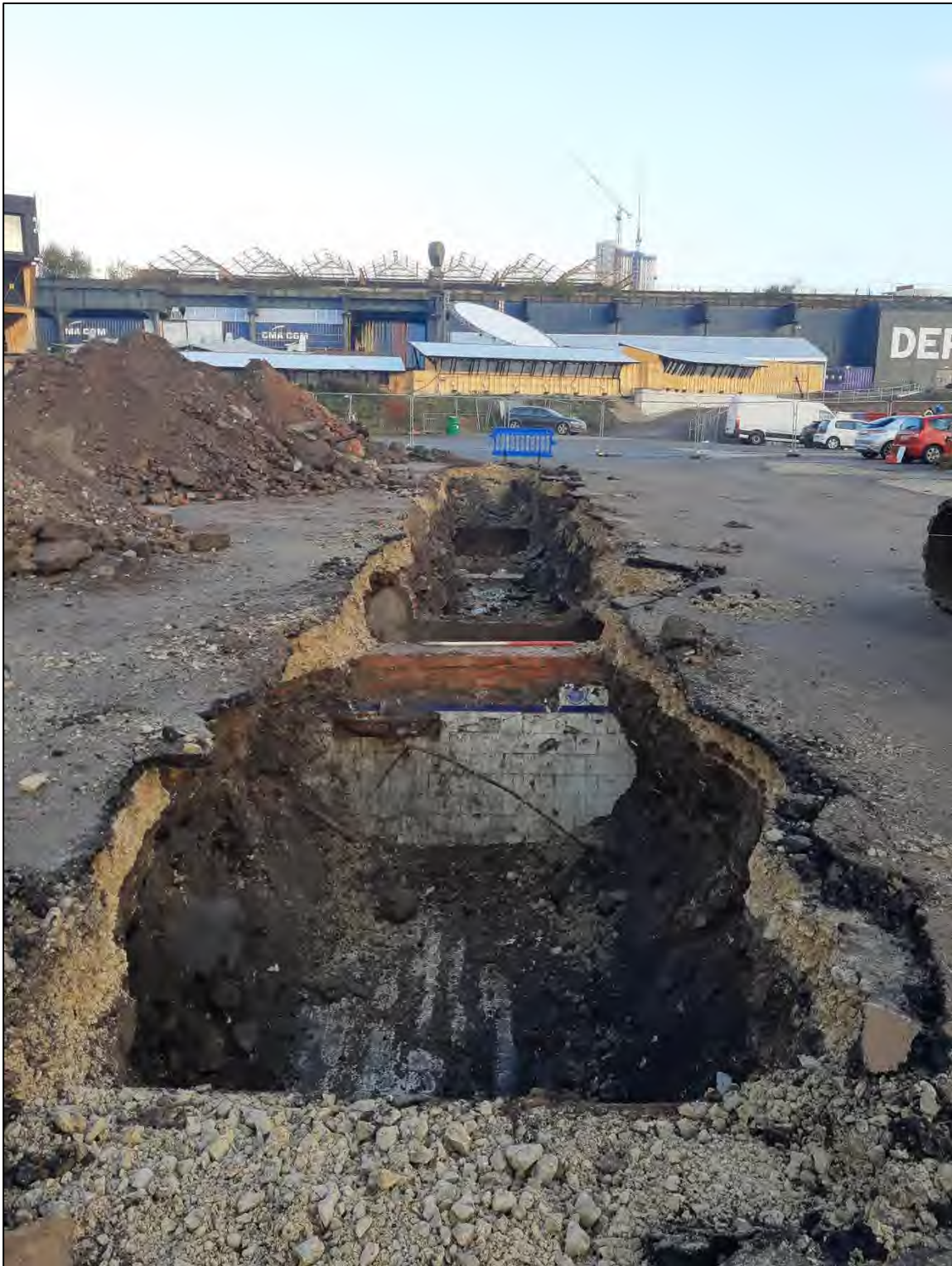
Plate 32: Trench 8, looking north.
