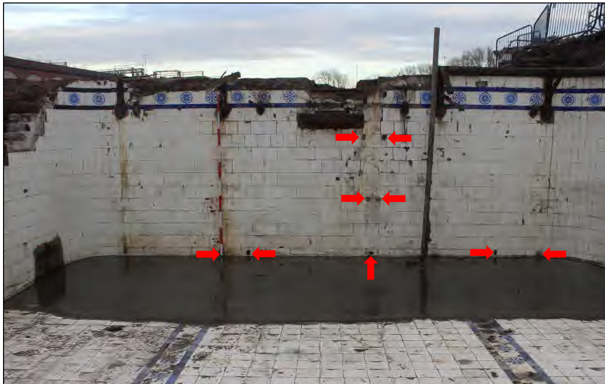
Plate 62: The eastern end of Pool 225 showing the position of the fixings for the steam injection pipe (removed) and L-shaped brackets visible above the waterline (2m scale)
