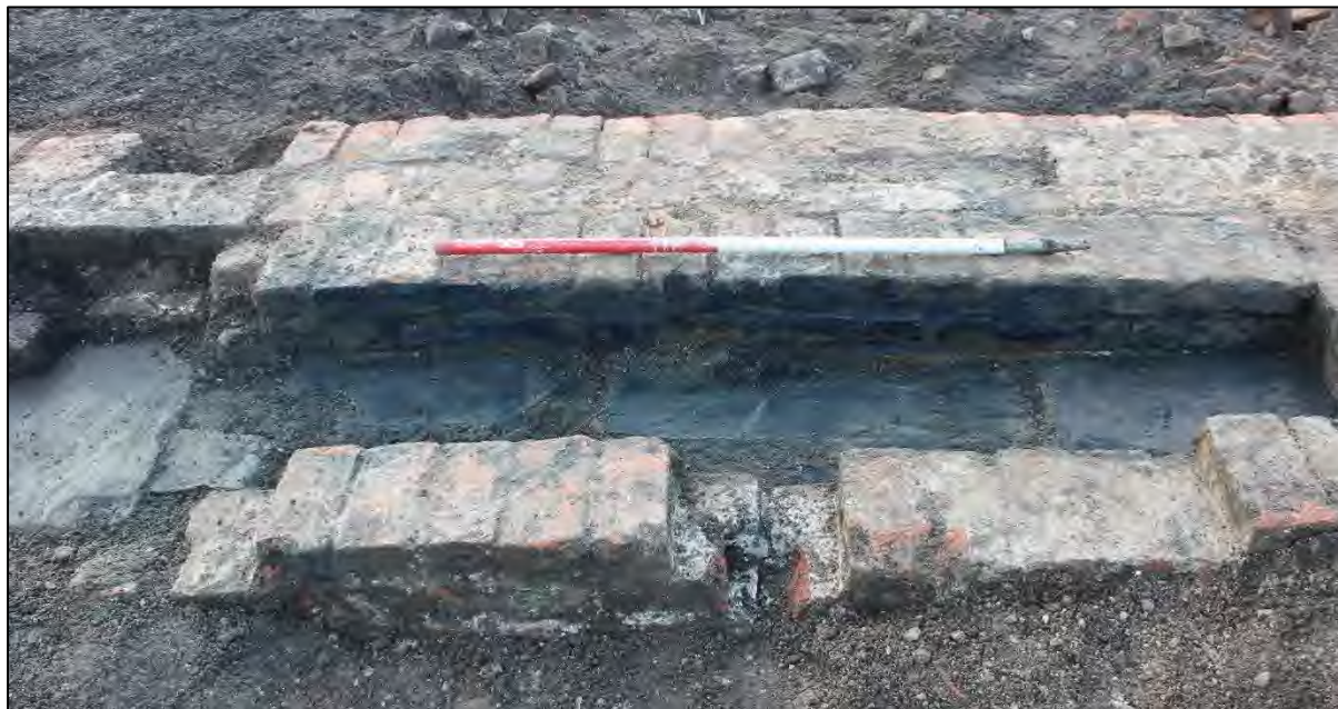
Plate 81: Slate-lined drain 3039 (1m scale)
