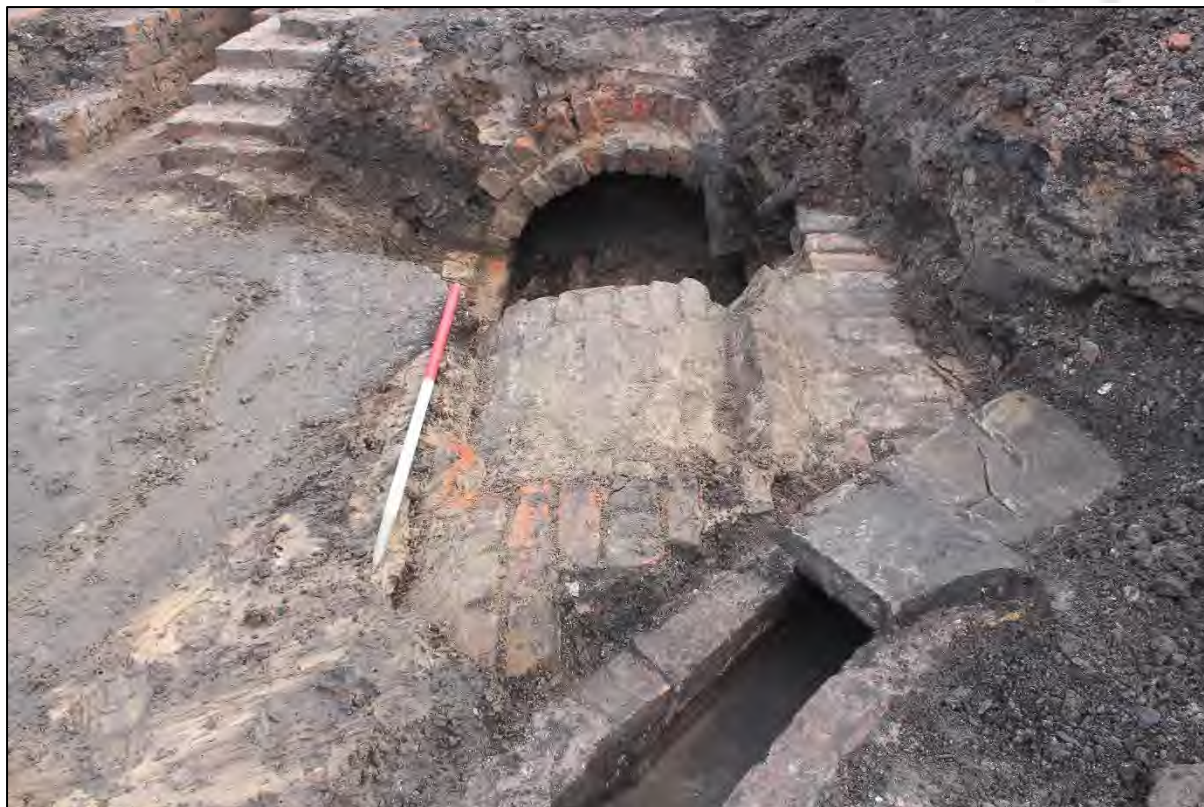
Plate 85: Vaulted culvert 3079 truncated by drain 3052
