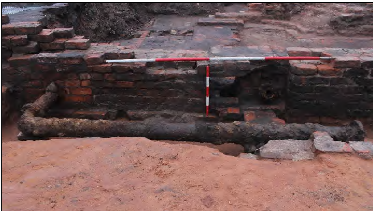
Plate 149: Eastern elevation of wall 3070 showing the blocked apertures in the wall (2m and 0.50m scales)
