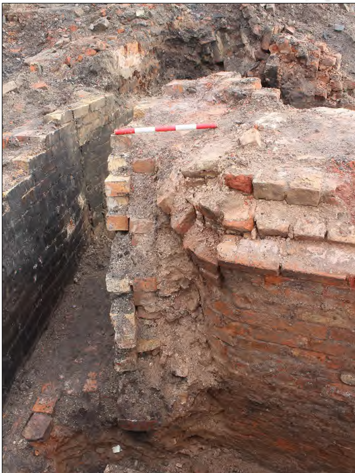
Plate 133: View of the junction between walkway 3069 and flue 3064, looking north-east (0.50m scale). Note the original handmade brick wall (unscorched) and surviving vaulting. This was altered by the infill of walkway, followed by the raising of the floor surface within flue 3069 and relining. The modified flue cut off access to the walkway.
