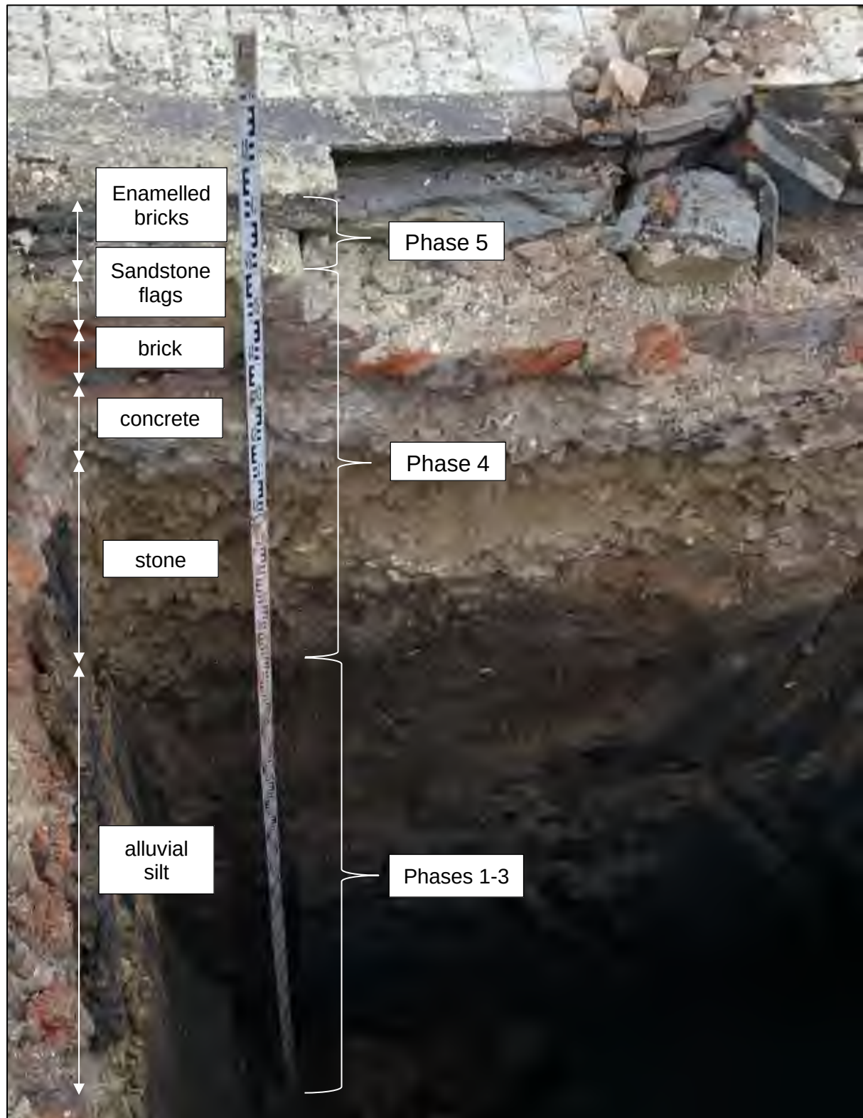
Plate 49: Sondage through the base of Pool 226 showing the composition of the foundations above earlier layers of alluvial silt
