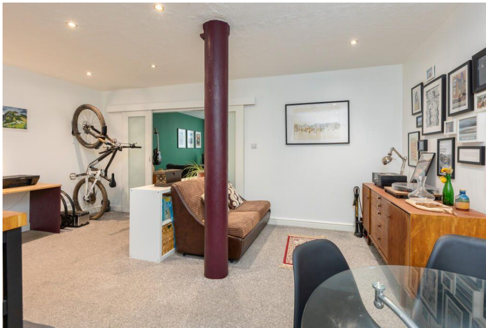
Figure 1 – Existing Cast Iron Column
