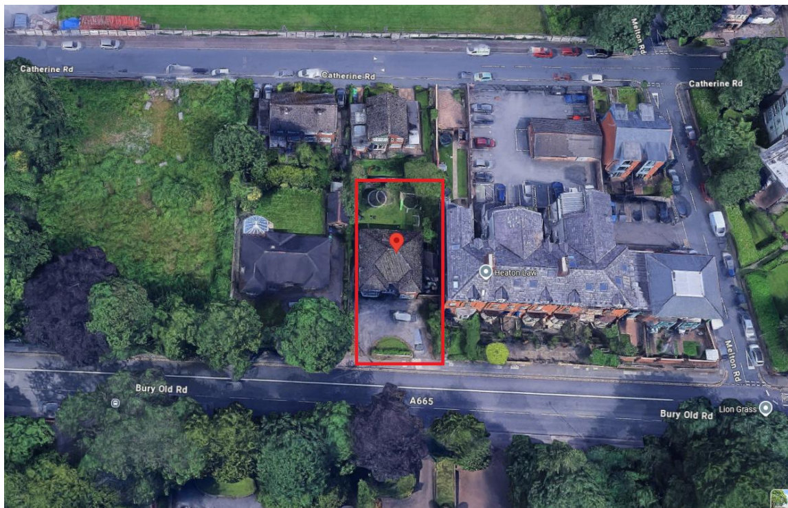
A view of the site from Google Earth
