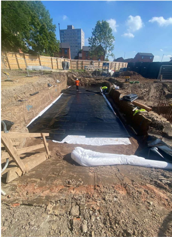
Figure 3 - Attenuation Tank A Installation
