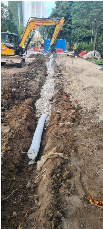
Figure 15 – Rain Garden installation
