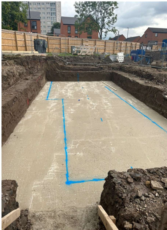
Figure 2 - Attenuation Tank A Installation
