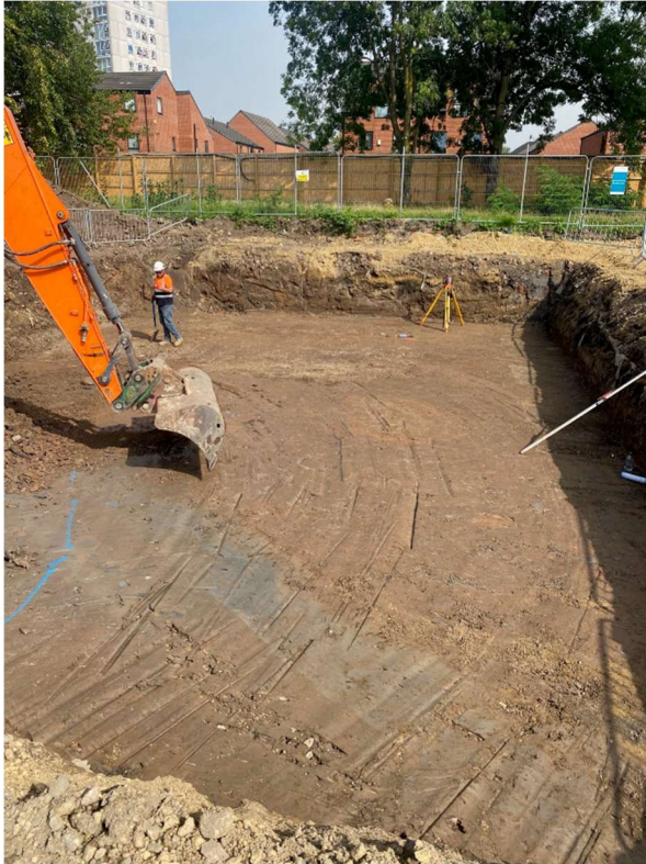
Figure 5 - Attenuation Tank B Installation
