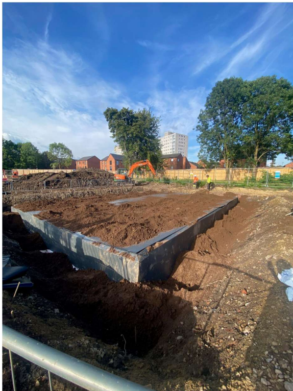
Figure 8 - Attenuation Tank B Installation
