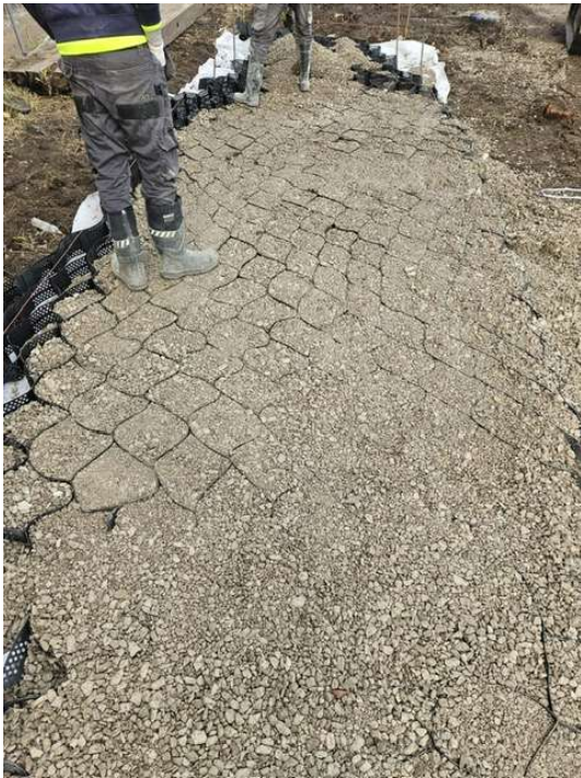
Figure 11 – Permeable Paving installation
