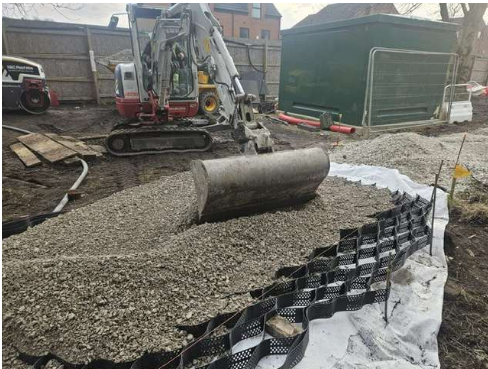
Figure 12 – Permeable Paving installation
