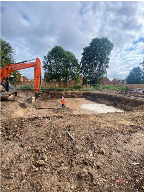
Figure 6 - Attenuation Tank B Installation
