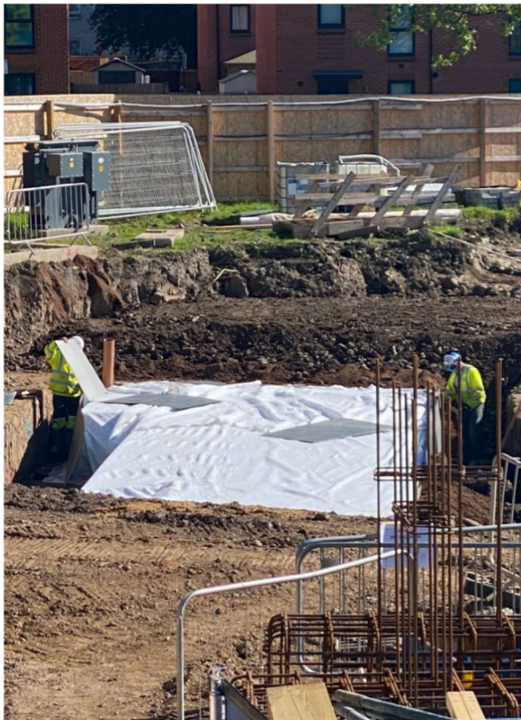
Figure 4 - Attenuation Tank A Installation
