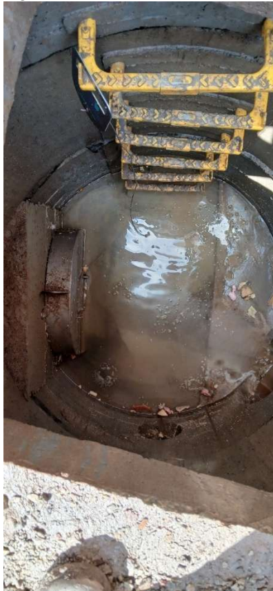
Figure 10 – Flow control Manhole S27 Installation
