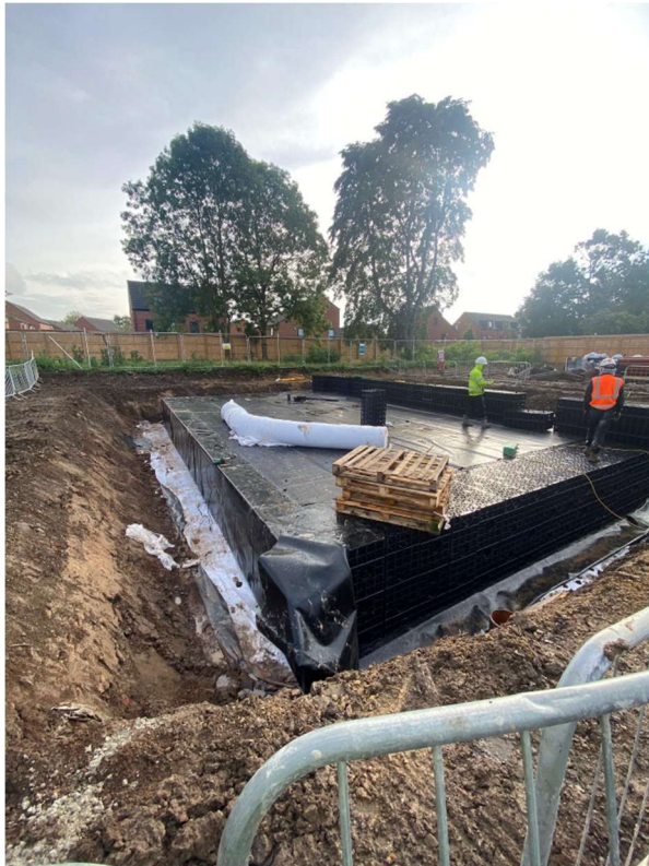
Figure 7 - Attenuation Tank B Installation
