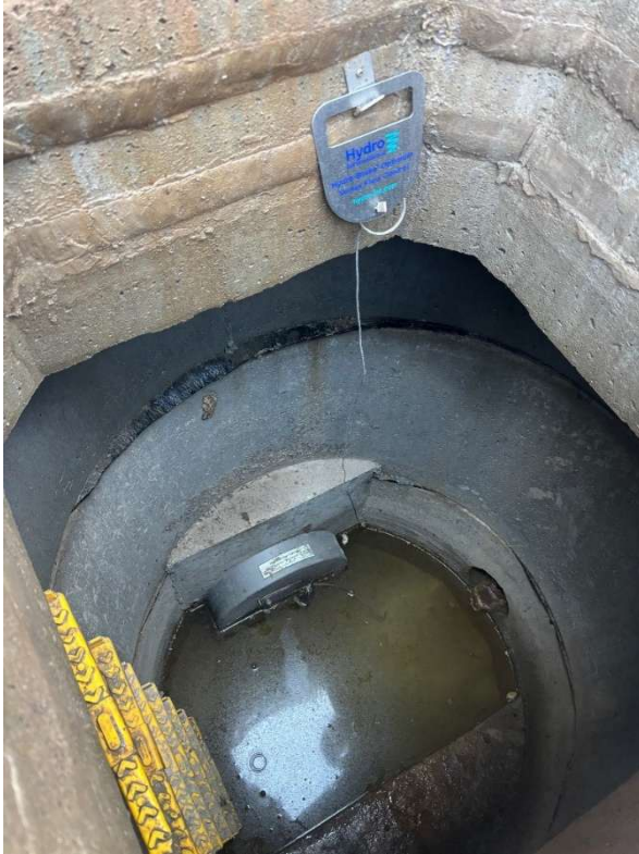
Figure 9 – Flow control Manhole S05 Installation
